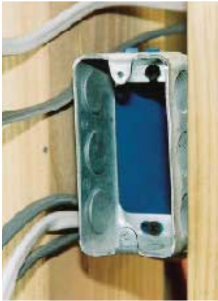
Figure 3. A box extension for single boxes (above) or two-gang boxes (right) can make up for differences in wall thickness.
