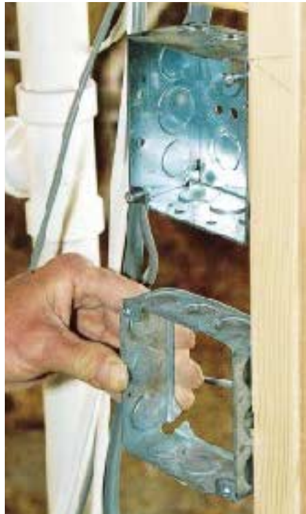
Figure 3. A box extension for single boxes (above) or two-gang boxes (right) can make up for differences in wall thickness.
