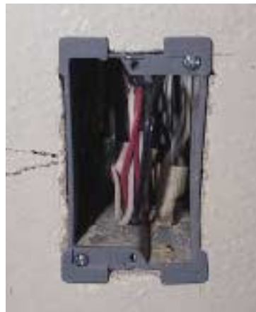
Figure 4. Remodel boxes and remodeler straps (left) are helpful for putting new boxes into old walls. Once in position, the flange on the front of the remodel box holds it firmly in place (right).
