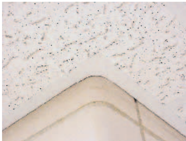
Figure 4. Factory-made trim pieces make neat work of outside corners.
