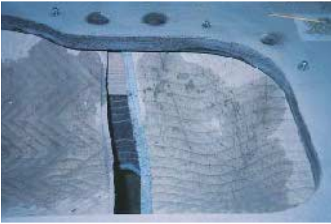
Figure 8. Undermount sinks are attached to stone countertops with clips that bolt into anchors. The anchors, which have female machine threads, are epoxied into shallow holes drilled in the stone.
