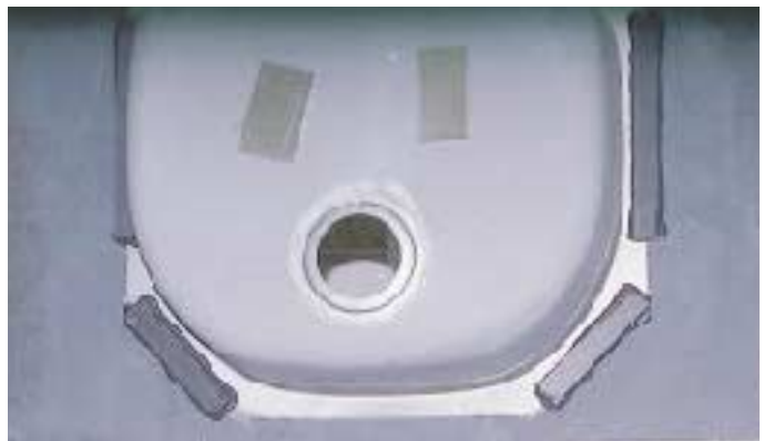
Figure 7. Some solid-surface fabricators attach undermount sinks with custom sink clips made from blocks of solid-surface material. The blocks are attached with solid-surface adhesive.
