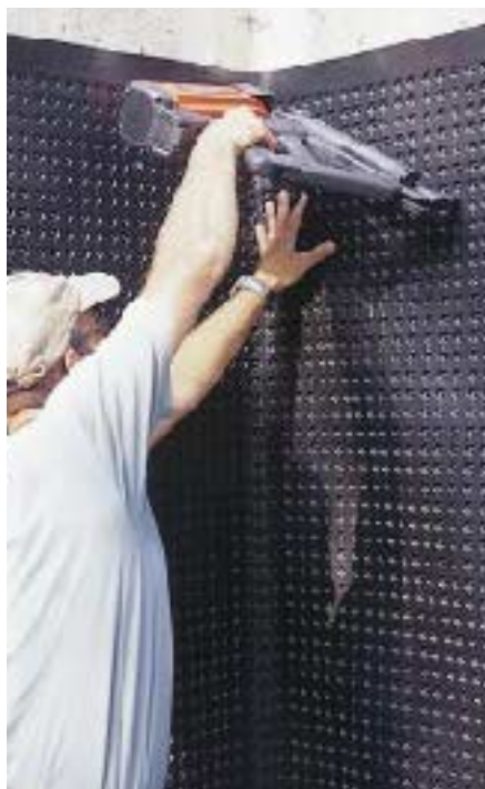
Figure 6. Similar to Delta-MS, the System Platon air-gap membrane can also be installed with the TrakFast.
