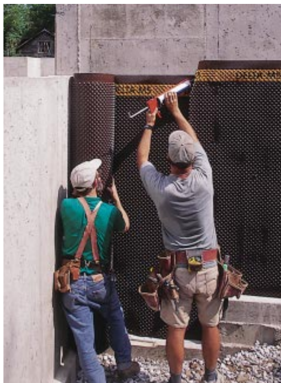
Figure 4. At joints, the dimples of the overlapping membrane nest in the dimples of the bottom sheet. A butyl caulk provides a seal.
