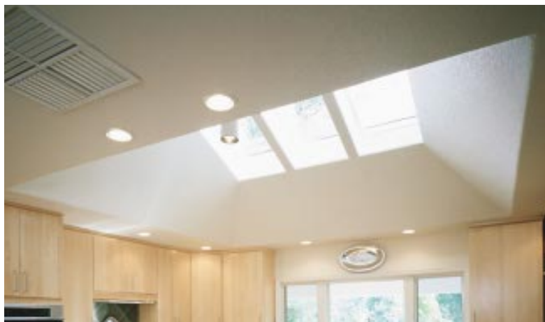
Figure 2. Before remodeling, this ranch kitchen felt dark and cramped, in spite of its 8-foot ceiling. The flared skylight shaft acts as a giant ceiling coffer to admit light and define the space (above). Another option is to terminate a flared shaft within a square-sided coffer (left).
