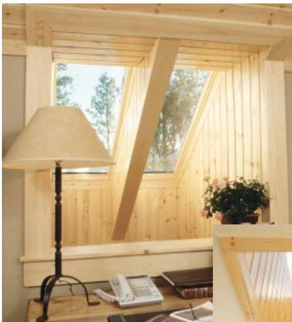
Figure 5. Ganged skylights admit daylight to the kitchen through a wood-paneled shaft (right). An opening to the study loft above the kitchen allows the same skylights to illuminate that space as well (above).
