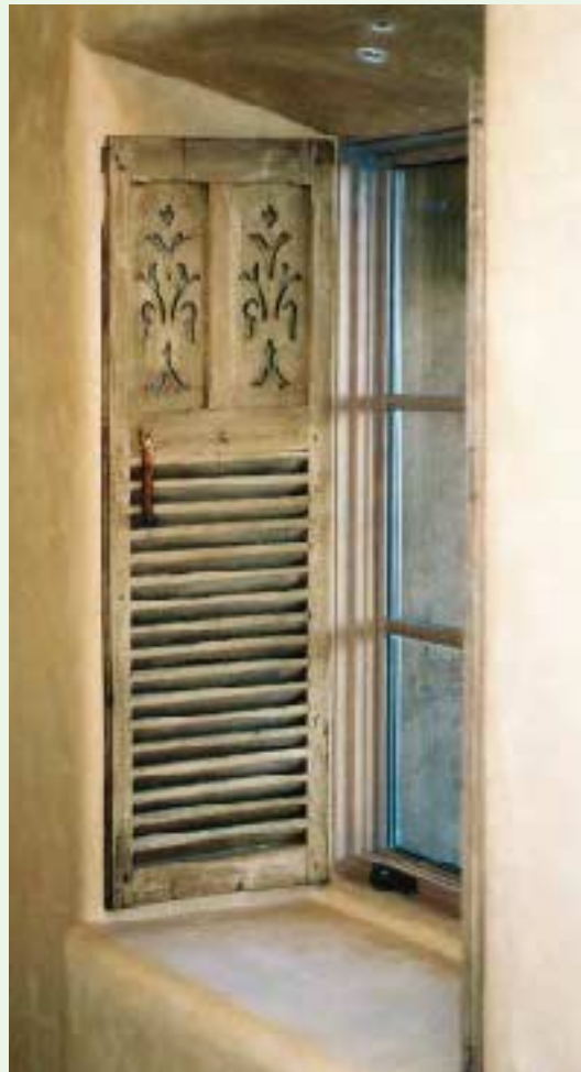
Figure B. Rastra walls provide thermal mass and lasting strength. Much of the architectural woodwork, including these shutters, was reused from other buildings.
