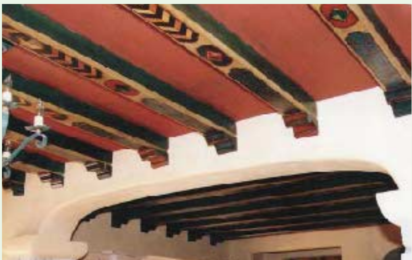
Figure D. Heavy timber reclaimed from an old railroad bridge was used throughout the house, including the great room (top). Salvaged, decorated beams were used in the kitchen and dining room (above).
