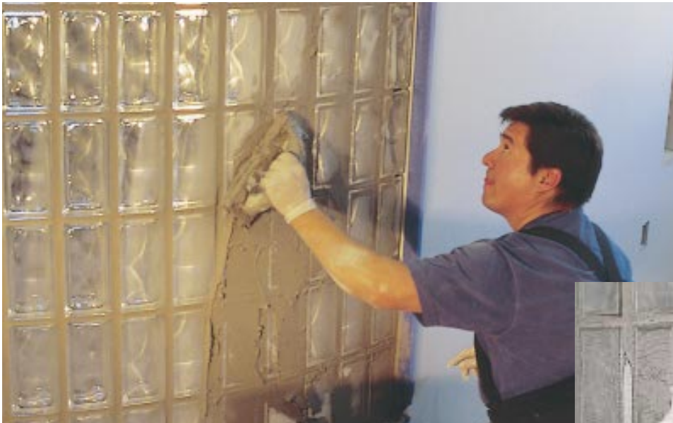
Figure 9. Sanded grout is applied evenly to the raked-out mortar joints.
