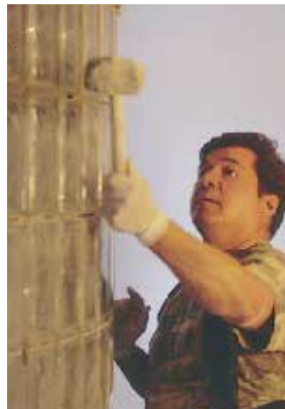
Figure 7. A rubber mallet is the tool of choice for making minor adjustments.
