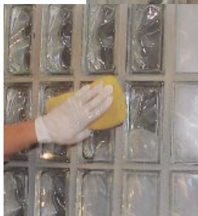
Figure 10. The author carefully wipes down the grout to get a dense, even finish. The haze is sponged off, leaving clean joint lines (inset).
