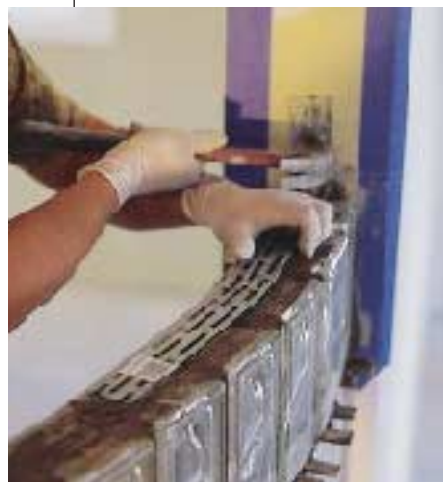
Figure 8. Every other course gets a panel anchor nailed to the wall with galvanized nails and embedded in the mortar.
