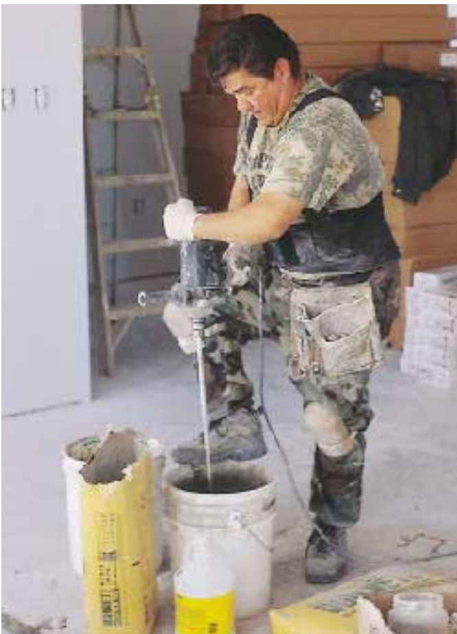
Figure 3. The author uses acrylic-fortified Quikrete mortar, which he mixes with an electric drill and paddle mixer.
