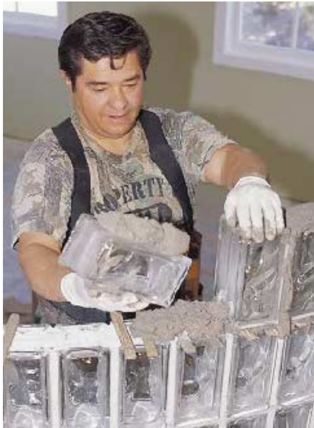
Figure 4. Wood spacers made from screen molding ensure consistent bed joints.
