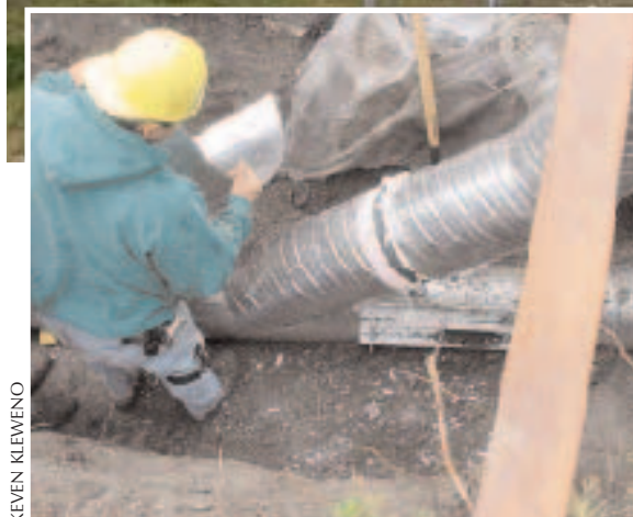
In rural Alaska, where permafrost is common, wastewater is often conveyed through above-ground pipes for disposal in sewage lagoons (above). Even when pipes can be buried, they are always encased in a thick layer of insulation (left).
