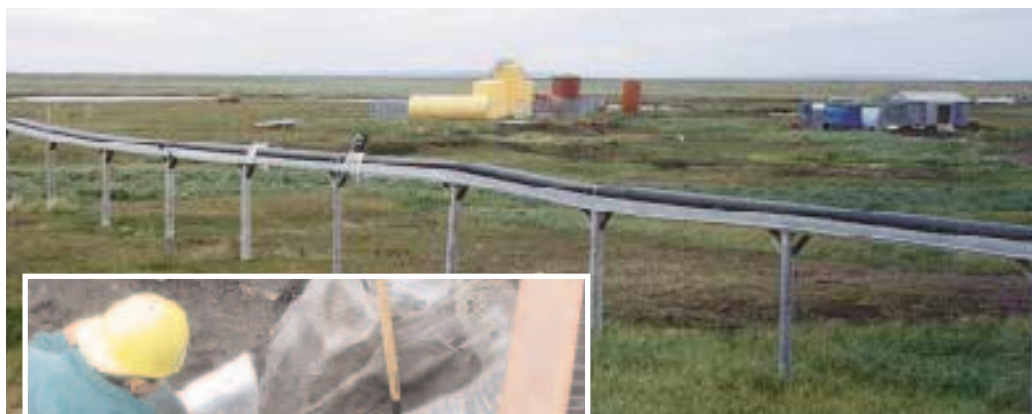
In rural Alaska, where permafrost is common, wastewater is often conveyed through above-ground pipes for disposal in sewage lagoons (above). Even when pipes can be buried, they are always encased in a thick layer of insulation (left).
