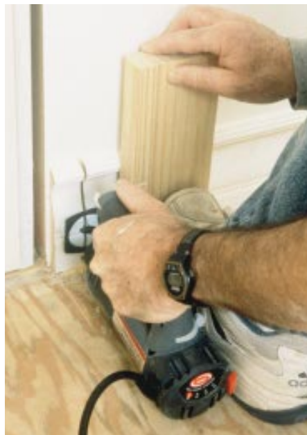
Figure 2. The RotoZip worked great for cutting baseboard in place (left) and ripping a window stool in place (right) without damage to surrounding materials.
