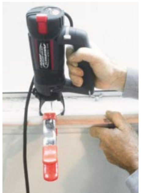
Figure 2. The RotoZip worked great for cutting baseboard in place (left) and ripping a window stool in place (right) without damage to surrounding materials.
