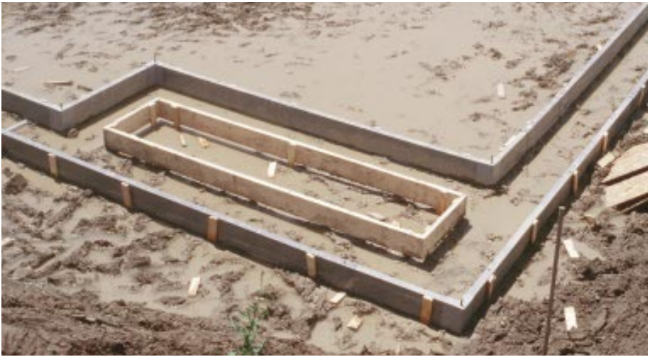
Figure 1. Vinyl Form-A-Drain footing forms stay in place as permanent drain pipes after the concrete sets.
