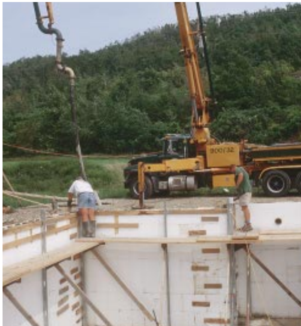
Figure 8. A pumper truck is essential for placing concrete in ICFs.
