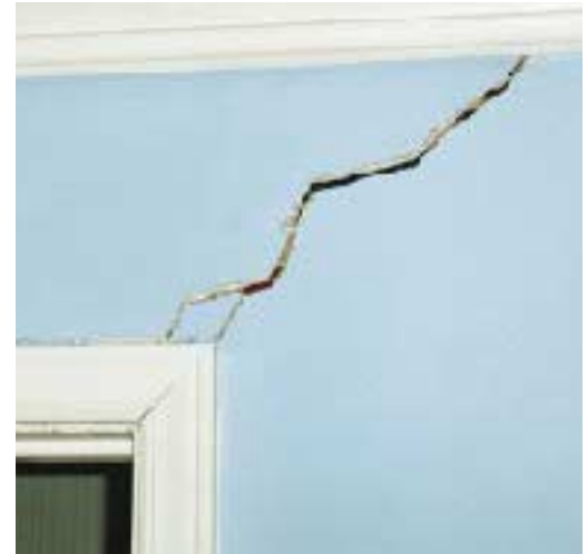
AMERICAN FOUNDATION & DRAINAGE
