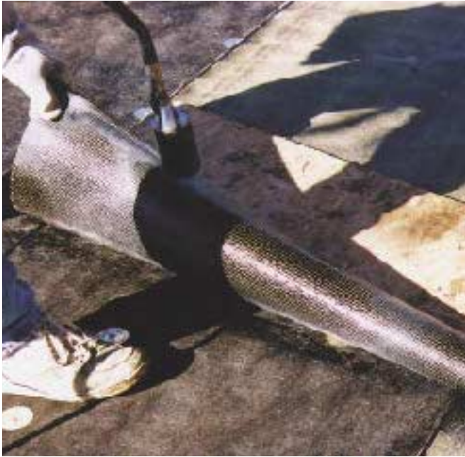
Figure 2. The bottom surface of the waterproof membrane has a coating that changes appearance when the correct temperature has been reached (left). Squeeze-out provides confirmation that the seam has properly fused (above).
