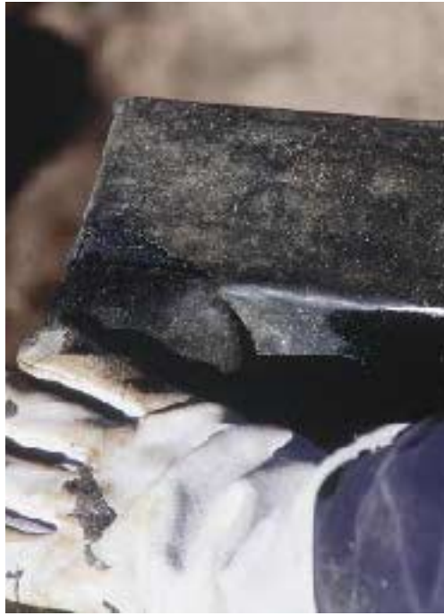
Figure 5. Because it can be cut and folded (far left), then heat-fused (left), torchdown is well suited for typically troublesome flat roof details like this inside parapet corner.
