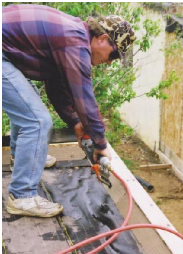
Figure 4. Fire-retardant cant strips ease the transition of the membrane up this short parapet, and also help prevent any sawdust inside the parapet wall from igniting during installation.
