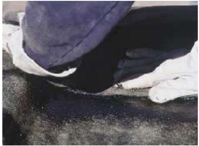
Figure 2. The bottom surface of the waterproof membrane has a coating that changes appearance when the correct temperature has been reached (left). Squeeze-out provides confirmation that the seam has properly fused (above).
