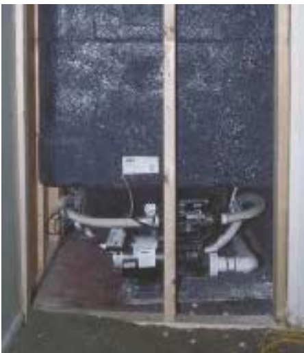
Figure 6. The pump is located at the foot of most whirlpool tubs. As long as the location is not blocked by a chimney or other obstruction, it's the best place for the access panel.
