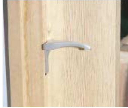
Casement windows have either exposed (left) or concealed (right) sash latch mechanisms.
