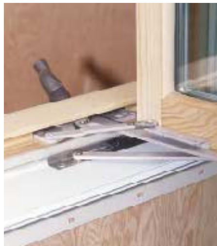
Routing the jamb and stool for the hardware leaves thin sections of wood in these locations on some windows.
