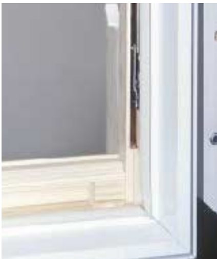
Routing the jamb and stool for the hardware leaves thin sections of wood in these locations on some windows.
