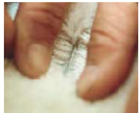
Figure 2. The visibility of a carpet seam depends on many factors, including the type and regularity of the face tufting. Irregular tufting rows force seam cuts to wander, making a true edge match impossible. Textured, berber styles are notoriously difficult to seam.
