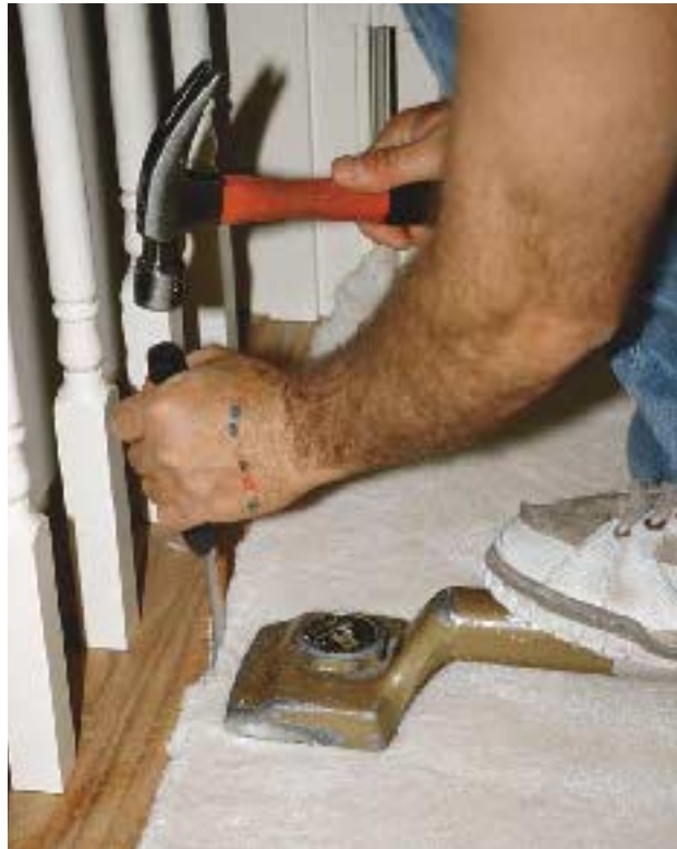
Figure 1. Finished wood thresholds and grounds at balustrades and stair railings provide a neat transition and involve less carpet installation labor.
