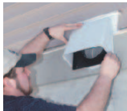
Figure 8. An HRV system requires two exterior ports, an intake port and an exhaust port. These identical 6-inch ports are protected by vent hoods and are usually located at the rim joist.
