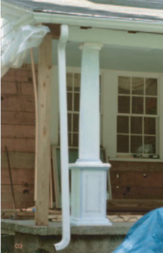
Figure 1. Sometimes scale drawings are not enough: A mock styrofoam column helped the clients visualize what they were getting (above). In the final design (right), manufactured cedar columns sit atop a basic MDO box pedestal trimmed with Honduras mahogany stiles and rails and stock moldings to imitate true raised panels.
