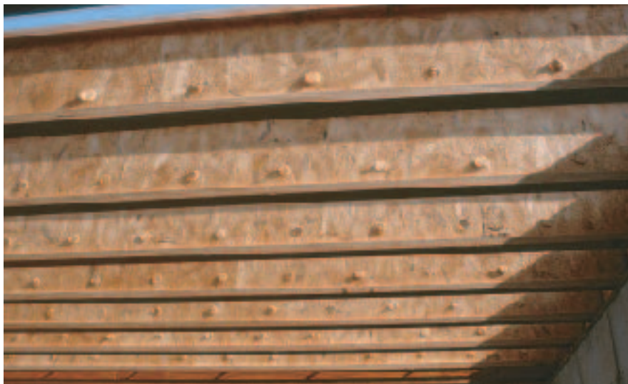
Figure 9. Taking advantage of the utility knockouts is a secondary consideration to maximizing materials. When it's practical, cutting joists from the factory end ensures automatic hole alignment for cross-joist wiring or plumbing runs, but in the effort to maximize materials, this is not always possible.
