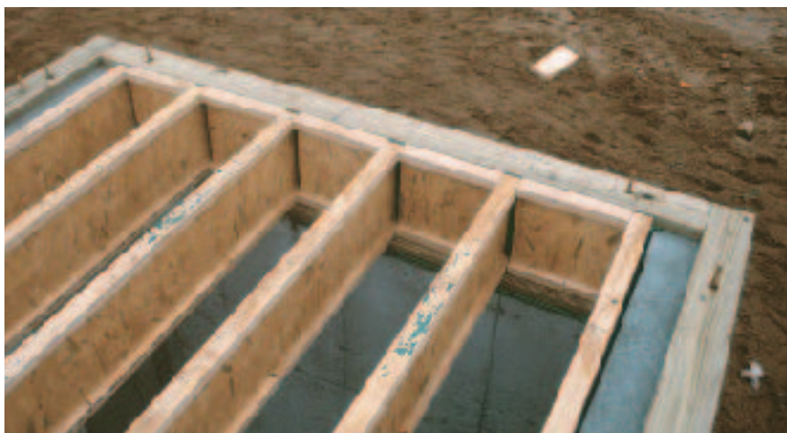
Figure 7. Pressure blocking holds the joists upright on a recessed, inset mudsill.
