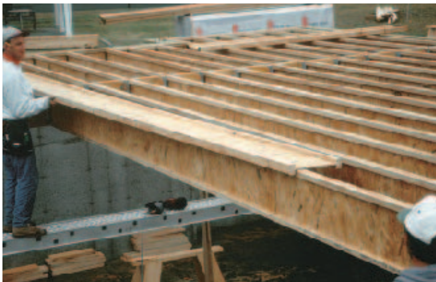
Figure 6. The floppiness of a long I-joist is controlled by feeding it out along the edge of the preceding member to the opposite side.
