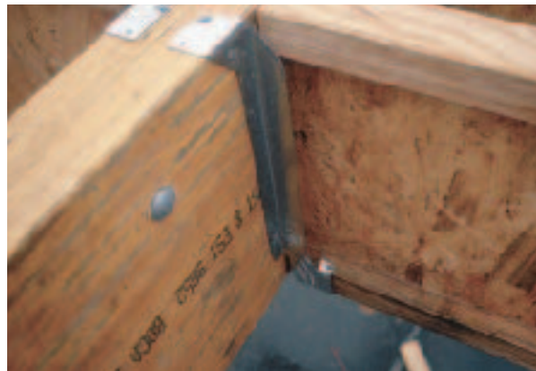
Figure 3. The joist hangers used by the author have a bendable tab that wraps the bottom flange of the I-joist, preventing movement.
