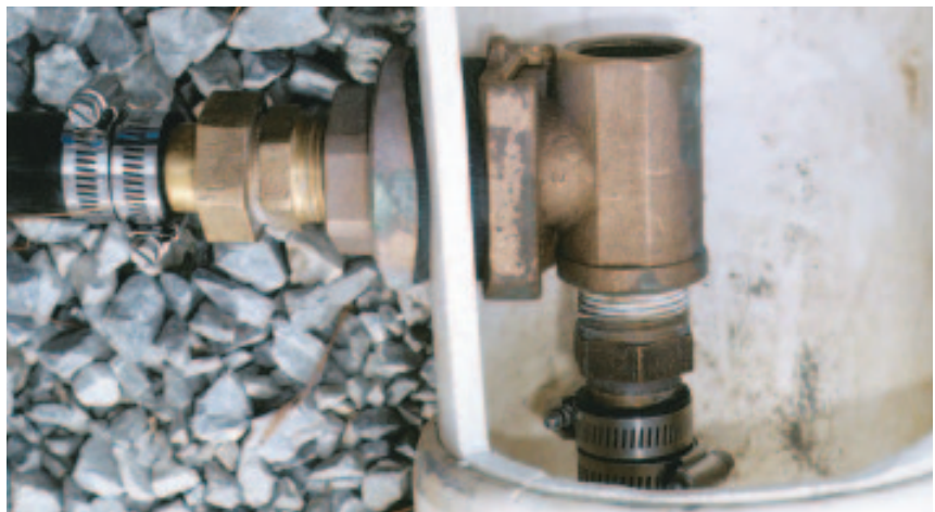
Figure 9. The two-piece pitless adapter connects the pipe from the house to the pipe running to the pump. The piece on the left in the top photo is mounted on the well casing below the frost line; the piece on the right is slid onto its mate and allows the pump to be removed, if necessary. The O-ring seals the two pieces together. A little grease prevents damage to the O-ring as the two are joined. The female threads at the top of the assembled pitless adapter (bottom) receive the homemade T bar, which lowers it to its mate mounted to the well casing.
