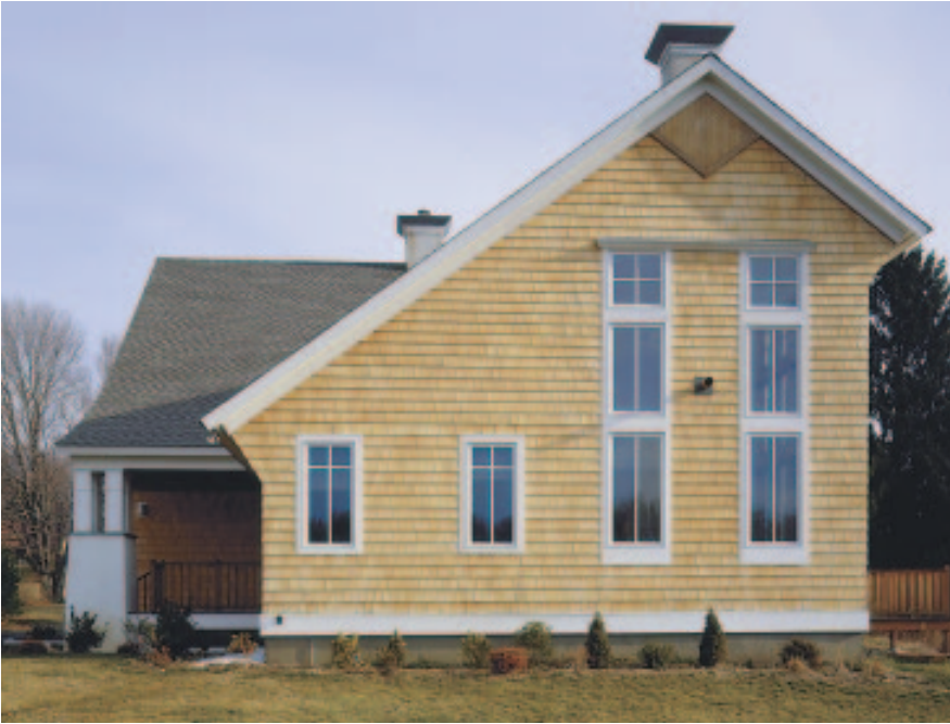
Figure 5. An ornamented peak and projecting “rooflet” over the stacked windows adds a sense of unity to a side elevation that might otherwise seem disorganized and chaotic.
