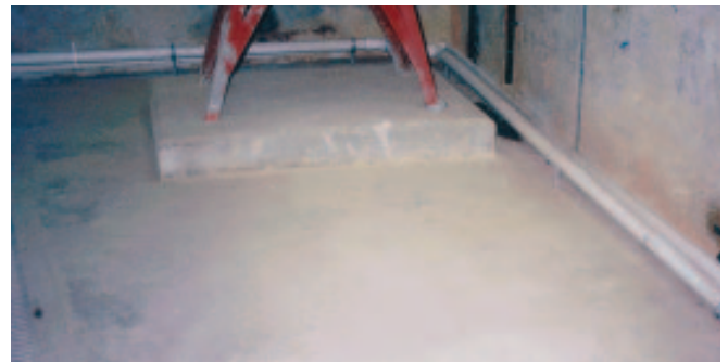
The dry basement after electronic treatment, with no additional drainage.
