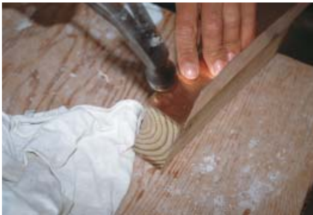
Figure 8. Copper drip cap adds a nice touch to the completed homes. It's cut about an inch longer than the head casing and bent over the ends with a hammer on a block of scrap wood (above). The completed cap is slid up behind the housewrap when the frame is installed (left).
