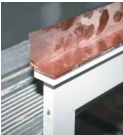
Figure 8. Copper drip cap adds a nice touch to the completed homes. It's cut about an inch longer than the head casing and bent over the ends with a hammer on a block of scrap wood (above). The completed cap is slid up behind the housewrap when the frame is installed (left).
