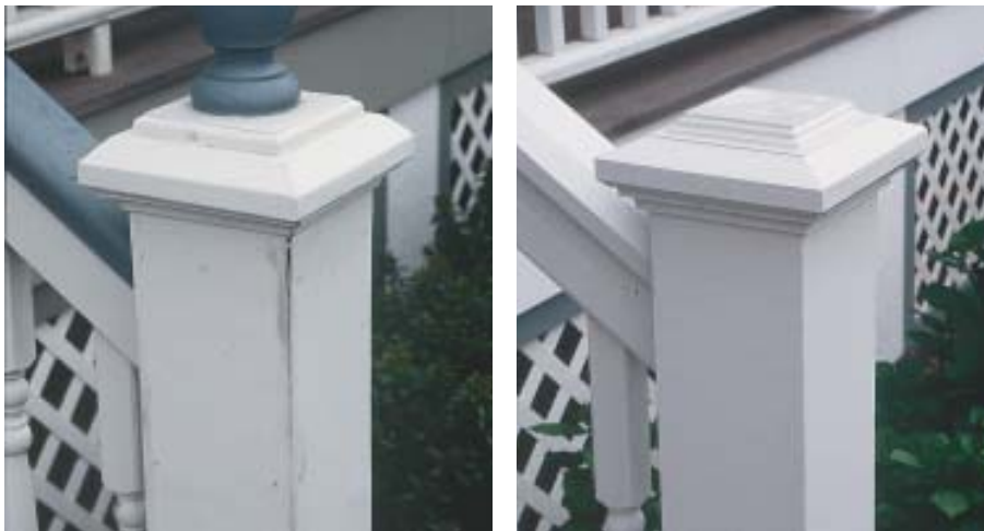
Figure 1. This hardboard product started showing signs of swelling after a year, even though the manufacturer's installation instructions were carefully followed (left). The Azek's PVC composition has held up better and still looks good three years after installation (right).
