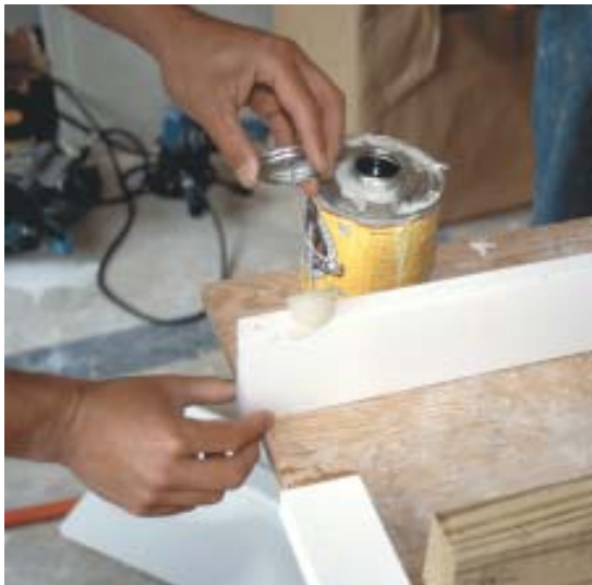
Figure 4. PVC cement actually fuses corners together. This keeps corners tight and eliminates a possible source of water infiltration. Joints must be held together tightly with nails or screws while the glue sets, because the cement can't bridge gaps like other adhesives.
