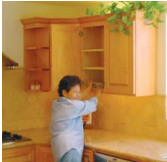
Figure 2. At 16 inches above the countertop, the tops of the wall cabinets were displayed and the client's access remained limited by her reach, so the author maintained a standard 18-inch spacing above the countertop and focused on base cabinet storage.
