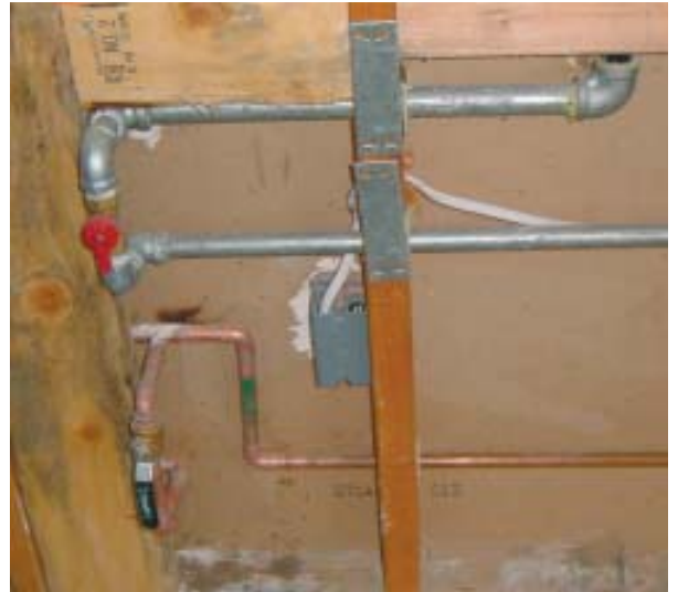
Figure 3. The author relied on full-extension drawer storage for pots, pans, and dishes and relocated the microwave from above the range to the island cabinet (left). The gas shutoff valve, installed in the back of an adjacent cabinet, allows the cooktop to be strapped in for earthquake-proof stability. A ball-valve shutoff on a dedicated water line for a pot-filler spigot and the refrigerator's icemaker shares the same cabinet (right)
