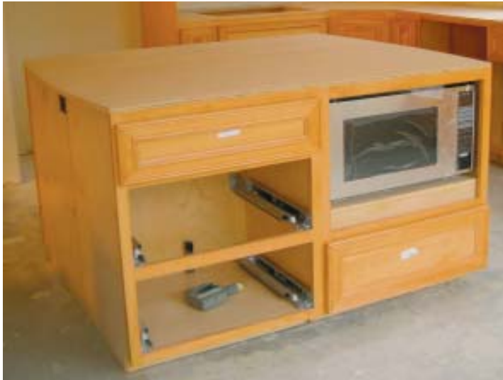
Figure 3. The author relied on full-extension drawer storage for pots, pans, and dishes and relocated the microwave from above the range to the island cabinet (left). The gas shutoff valve, installed in the back of an adjacent cabinet, allows the cooktop to be strapped in for earthquake-proof stability. A ball-valve shutoff on a dedicated water line for a pot-filler spigot and the refrigerator's icemaker shares the same cabinet (right)
