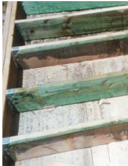
Figure 4. Joists that are too far gone to repair must be replaced between the wall plate and the new double rim joist (left). The rim hangs at the ends of the intact cantilevered joists on upside-down joist hangers. The replaced “cripple joists” are hung conventionally (right).
