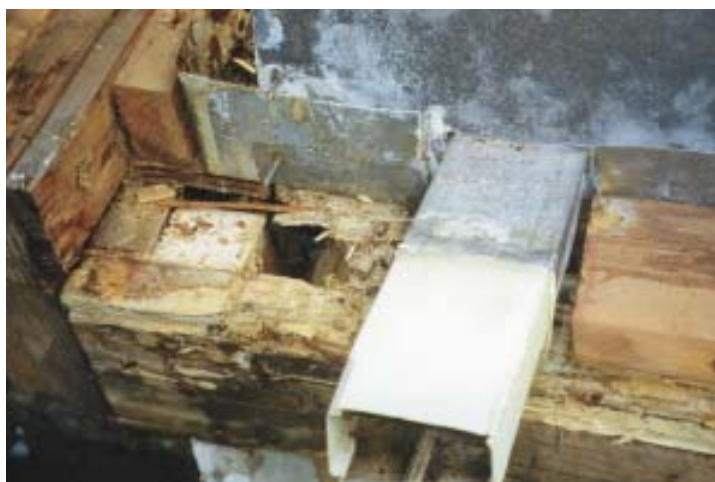
Figure 2. Improperly flashed scuppers (left) and floor drains (right) often allow water into the framing, leading to hidden rot.
