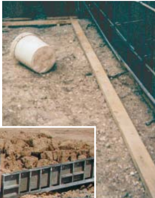
Figure 4. The bases of the wall forms rest atop 2x4s nailed to 2x4 stakes driven into the soil at approximately 2-foot intervals. At right, one form has been erected and braced, and the rebar has been wired in place. After cardboard void forms have been placed at the bottom of the wall, the second form will be erected. Below, void forms and rebar are test-fitted before the forms are erected.
