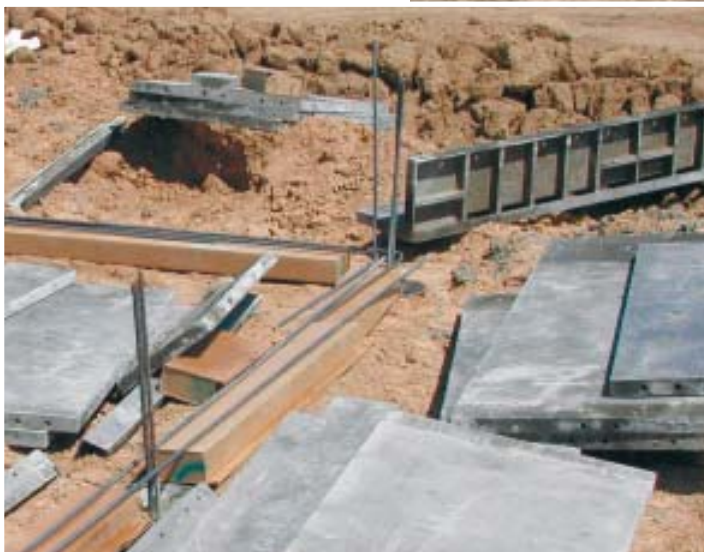
Figure 4. The bases of the wall forms rest atop 2x4s nailed to 2x4 stakes driven into the soil at approximately 2-foot intervals. At right, one form has been erected and braced, and the rebar has been wired in place. After cardboard void forms have been placed at the bottom of the wall, the second form will be erected. Below, void forms and rebar are test-fitted before the forms are erected.
