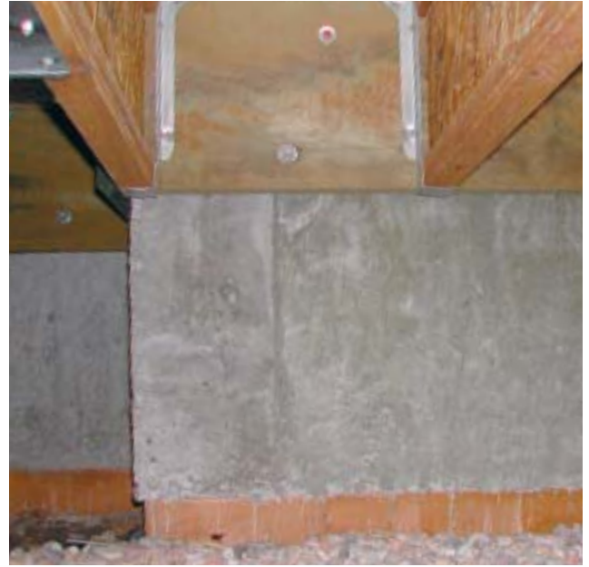
Figure 8. Steel saddles, expansion-bolted to the foundation walls, support the ends of the central girder in the crawlspace (above). The ends of the I-joists rest in joist hangers fastened to pressure-treated ledgers (right).
