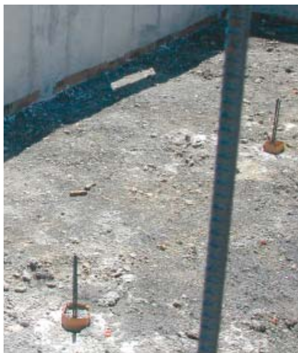
Figure 6. In a top view into the forms just before the concrete pour, the void forms are visible at either side of the caisson at center (above). The vertical strands of rebar extending from the caisson will anchor the foundation wall to the caisson, which will bear the structure’s weight. After the forms have been stripped, the edges of the void forms are visible at the base of the wall, except where interrupted by caissons (left).
