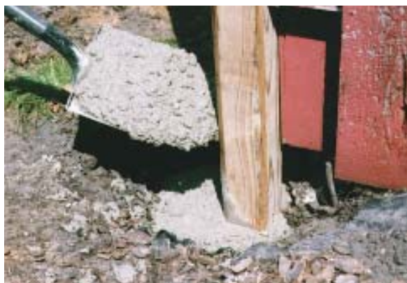
Figure 4. A replacement post is nailed to an adjacent fence section and plumbed with temporary bracing as site-mixed concrete is poured around the base (above). Bringing the concrete up to grade protects the post from rot where it is most vulnerable (left).
