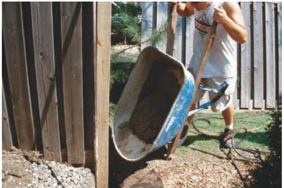
Figure 4. A replacement post is nailed to an adjacent fence section and plumbed with temporary bracing as site-mixed concrete is poured around the base (above). Bringing the concrete up to grade protects the post from rot where it is most vulnerable (left).
