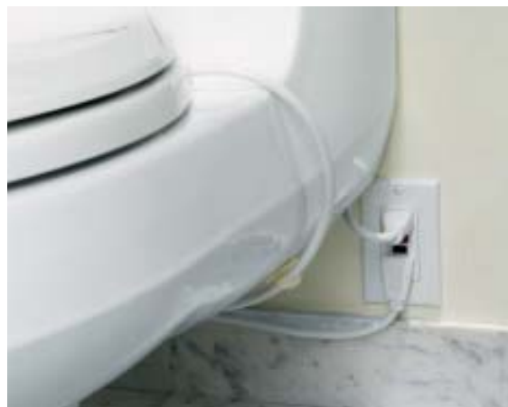
Figure 5. Kohler's Power Lite series of toilets contain compact submersible pumps that are said to produce a flush similar to that of a pressure-assisted fixture. A GFCI-protected outlet is required to supply power to the pump.
