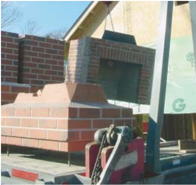
The 36-inch-wide by 30-inch-tall by 23-inch-deep firebox is lifted from the truck. The design includes a 60-degree throat slope and a rounded smoke shelf for increased performance. A built-in ash dump, with a removable drawer, is located below the firebox.
