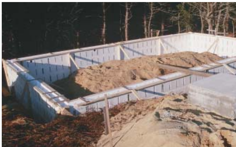
Figure 5. Vertical 2x4 braces spaced about 8 feet on-center tie into a 2x4 "ladder" laid over the top of the forms to stiffen them. Diagonal braces run from the vertical braces back to the ground (above), and a working platform tied into the bracing system provides easy access to the tops of the forms (right). It's important to use at least the minimum bracing specified in the manual.
