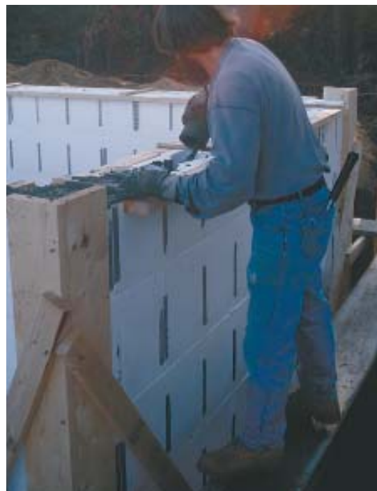
Figure 5. Vertical 2x4 braces spaced about 8 feet on-center tie into a 2x4 "ladder" laid over the top of the forms to stiffen them. Diagonal braces run from the vertical braces back to the ground (above), and a working platform tied into the bracing system provides easy access to the tops of the forms (right). It's important to use at least the minimum bracing specified in the manual.
