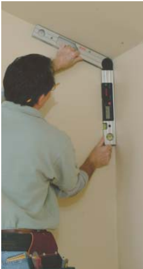
Figure 6. To figure the miter angle for the bottom end of the rake molding, the author first measures the ceiling-wall angle (above), then uses basic geometry to solve for the cut angle.
