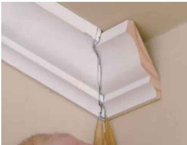
Figure 2. To cut the unusual scribes that are required when fudging an inside corner (above), the author uses a jigsaw fitted with a coping foot (above right), as well as a grinder (right), for making extra steep back bevels.
