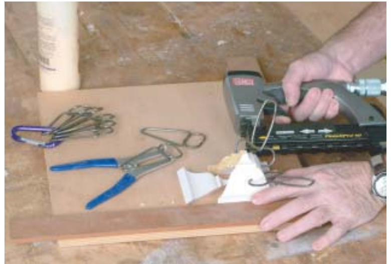
Figure 7. Pendants can provide a point of termination for crown molding and eliminate the need to join a rake run with a horizontal run (left). The author makes pendants from scraps, mitering four pieces together using spring clamps, glue, and pin nails (right).
