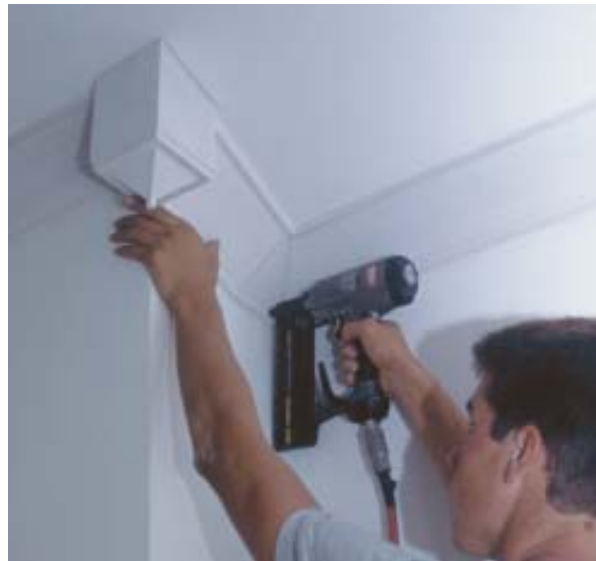
Figure 8. Pendants provide a ready solution for outside corners that interrupt a cathedral ceiling.
