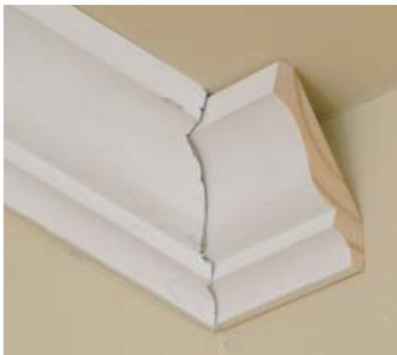
Figure 1. To “force” a crown molding corner on a cathedral ceiling, the author tips the molding on the horizontal run closer to plumb. That way, the height of the crown on the horizontal run more nearly matches the height of the crown coming down the rake, though the profiles will rarely match perfectly, especially on steeply sloped ceilings. Rebeveling the back of the crown at the bottom allows it to close tightly against the wall.
