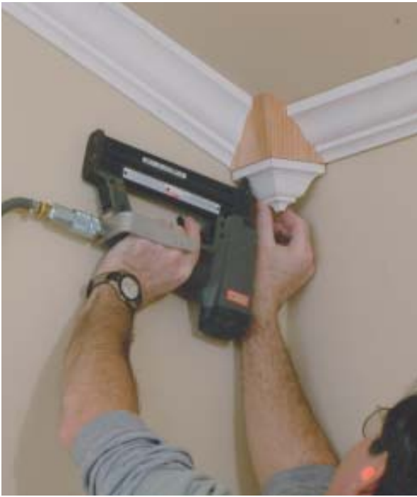
Figure 7. Pendants can provide a point of termination for crown molding and eliminate the need to join a rake run with a horizontal run (left). The author makes pendants from scraps, mitering four pieces together using spring clamps, glue, and pin nails (right).
