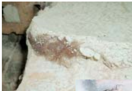
Horsehair used in old plaster may have been soaked with arsenic, making plaster demolition particularly harmful to remodelers.
