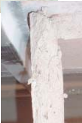
Horsehair used in old plaster may have been soaked with arsenic, making plaster demolition particularly harmful to remodelers.
