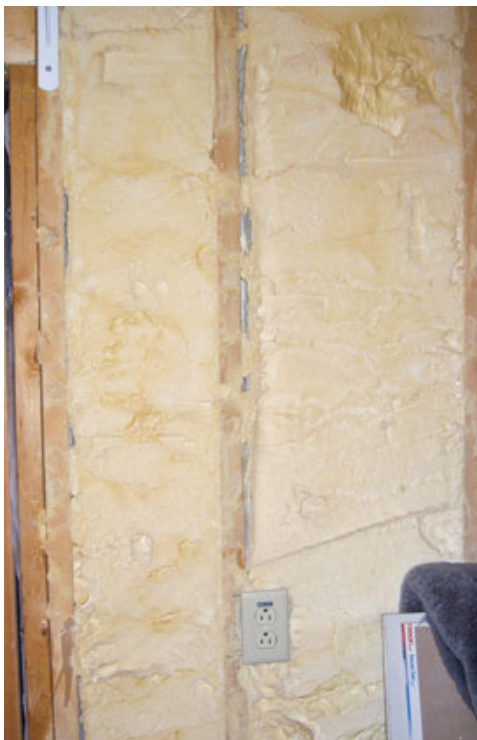
Figure 2. By taking surface and air temperature readings on both sides of the foam-insulated garage walls, the author was able to estimate the R-value of the insulation in that location and — by extrapolation — in the cathedral ceiling.
