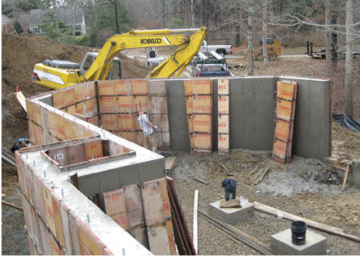
Figure 4. Slab areas were poured atop full-height foundation compartments. The smaller of the two compartments is visible on the left side of the photo at left; the larger, not yet complete, is defined by the row of vertical rebar visible at the rear. The finished compartments were filled with compacted soil (above) and later capped with concrete slabs, providing a code-required setback from the septic system's leaching field.
