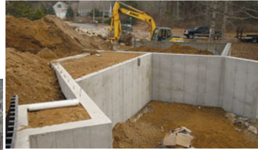
Figure 4. Slab areas were poured atop full-height foundation compartments. The smaller of the two compartments is visible on the left side of the photo at left; the larger, not yet complete, is defined by the row of vertical rebar visible at the rear. The finished compartments were filled with compacted soil (above) and later capped with concrete slabs, providing a code-required setback from the septic system's leaching field.
