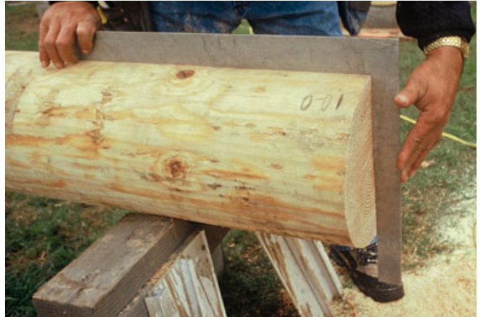
Figure 3. A framing square held to the “layout line” is used to mark the square cut at the end of the log (left). After making the cut, the carpenter checks for square (right), remembering to allow for any taper the log may have.
