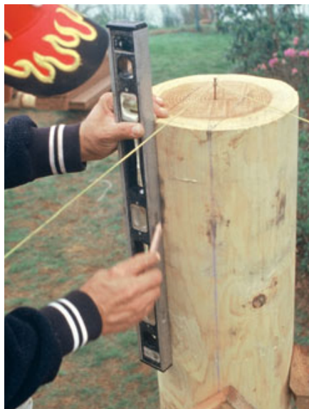
Figure 7. With the posts up and braced plumb, a string is used to establish the line of the beam. A carpenter uses a level to lay out the side cuts for the beam pocket (left), then makes the cutout with a chain saw (above), working off staging for stability.
