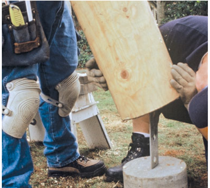
Figure 6. A torpedo level and a layout square are used to guide the drilling of holes for the anchor bolts (left). Placing the post is a two-person operation (right).
