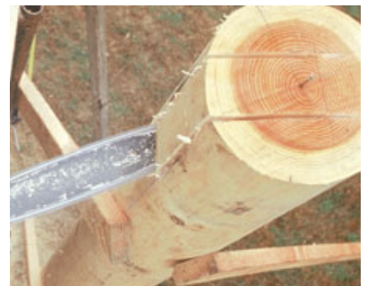
Figure 7. With the posts up and braced plumb, a string is used to establish the line of the beam. A carpenter uses a level to lay out the side cuts for the beam pocket (left), then makes the cutout with a chain saw (above), working off staging for stability.
