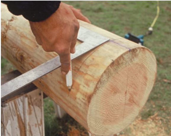
Figure 3. A framing square held to the “layout line” is used to mark the square cut at the end of the log (left). After making the cut, the carpenter checks for square (right), remembering to allow for any taper the log may have.
