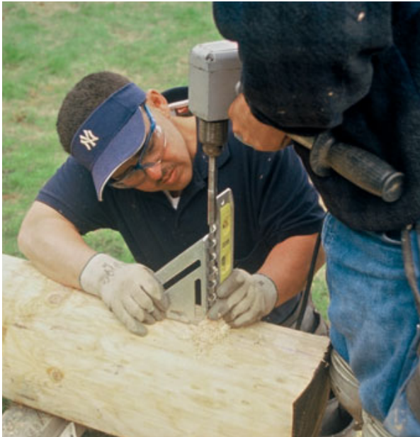
Figure 6. A torpedo level and a layout square are used to guide the drilling of holes for the anchor bolts (left). Placing the post is a two-person operation (right).
