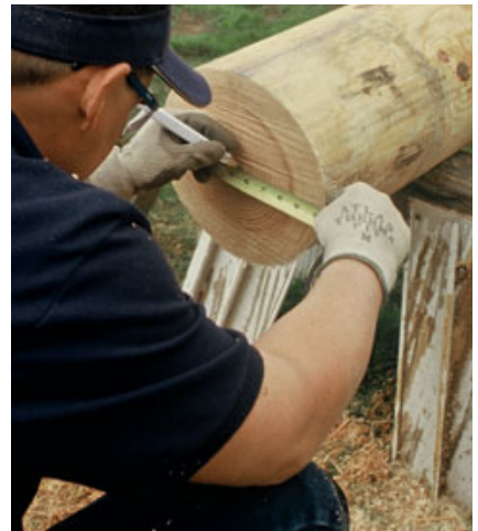
Figure 4. The hold-down anchor (above left) will fit in a slot cut in the post’s bottom. Anchors are rarely centered exactly on the pedestal, so the author carefully transfers the slot layout to ensure that the post will overhang the pedestal evenly.
