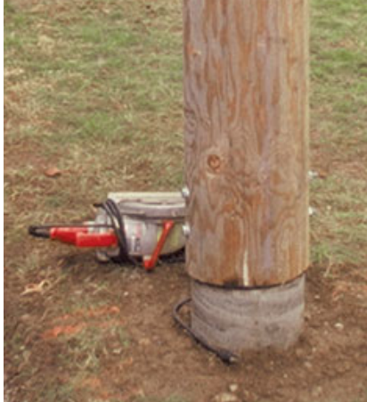
Figure 1. Because log posts are vulnerable to rot from water wicking up the end grain, the author makes the top of the footing 2 inches smaller than the post to provide a drip-edge.
