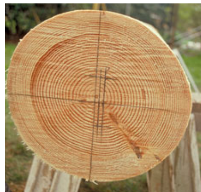
Figure 4. The hold-down anchor (above left) will fit in a slot cut in the post’s bottom. Anchors are rarely centered exactly on the pedestal, so the author carefully transfers the slot layout to ensure that the post will overhang the pedestal evenly.
