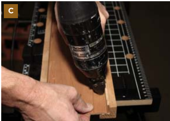
Figure 1. Newel construction starts with four 2x2 oak balusters with one corner ripped out. Plywood panels are glued with PL400 (A), then pinned in place (B). By using a plywood spacer while nailing the first panel to the second baluster (C, D), the author leaves room for the next perpendicular panel to slip snugly into place.
