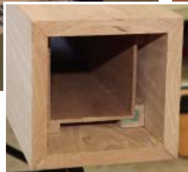
Figure 5. The newel is finished with a 12-inch-wide oak base, then capped and trimmed on site.
