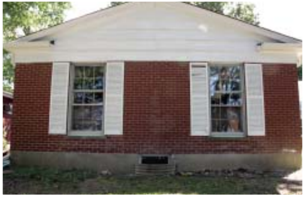
Figure 1. Although there was plenty of room for expansion in the basement area of this ranch, the small windows let in scant natural light and there was no means of egress (above). By adding the patio door and windows, the author made the interior space more livable and provided convenient access to the backyard and the lake beyond (right).
