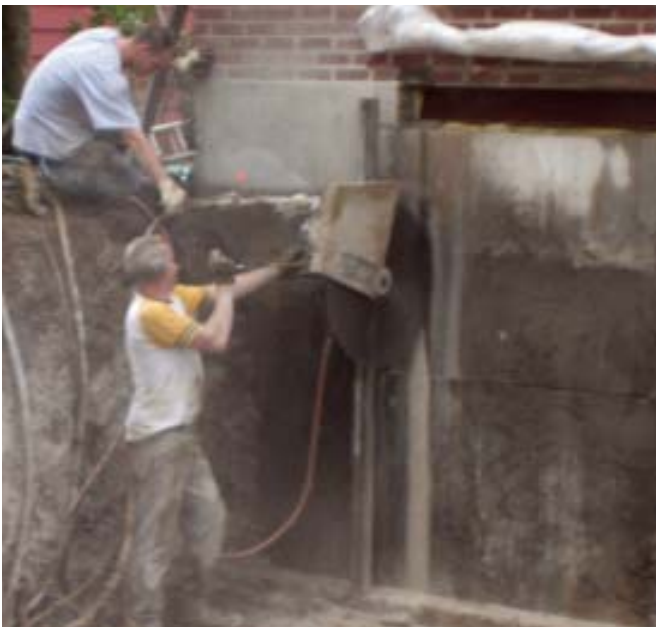
Figure 5. A day of excavating and grading left a flat, accessible site for the concrete-cutting subs. Once the opening was cut, the crew broke the concrete slabs into manageable pieces.
