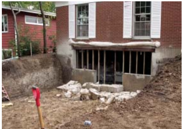
Figure 5. A day of excavating and grading left a flat, accessible site for the concrete-cutting subs. Once the opening was cut, the crew broke the concrete slabs into manageable pieces.
