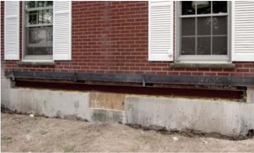
Figure 4. After slipping the I-beam into its slightly oversized pocket (above), the author shimmed it tight to the floor framing above (right). Before removing the temporary lintel, the missing course of brick was relaid.
