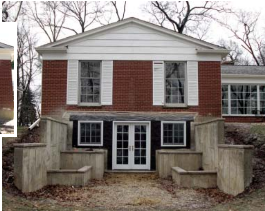
Figure 1. Although there was plenty of room for expansion in the basement area of this ranch, the small windows let in scant natural light and there was no means of egress (above). By adding the patio door and windows, the author made the interior space more livable and provided convenient access to the backyard and the lake beyond (right).
