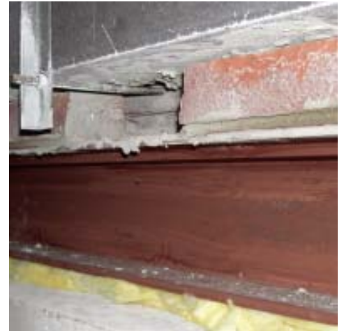
Figure 4. After slipping the I-beam into its slightly oversized pocket (above), the author shimmed it tight to the floor framing above (right). Before removing the temporary lintel, the missing course of brick was relaid.
