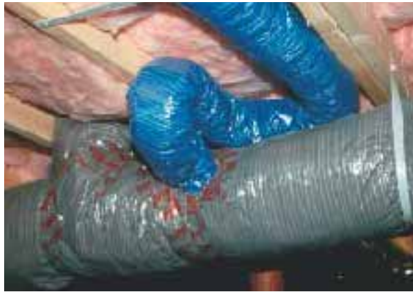
Figure 8. Branch ducts must be no shorter than 10 feet long and no longer than 25 feet. The flexi-duct can be coiled back upon itself to provide the minimum duct length, with no reduction in performance.
