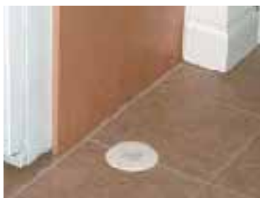
Figure 1. Continuously blowing outlets provide heating and cooling and can be installed high or low on the wall, as well as in the ceiling or floor. Placement isn't as important as providing an accurate number of outlets per room and avoiding blockage. The outlet grid design imposes laminar air flow, correcting noisy vents.
