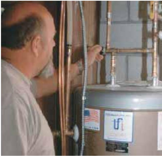
Figure 5. An operating temperature of 120° to 140°F permits use of a standard water heater to supply the fancoil unit. Slower passage of air over a larger than conventional coil surface enables higher coil-to-air heat transfer. Because of the lower temperatures, all ductwork must be completely insulated to retain operating efficiency.
