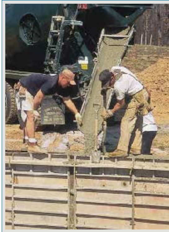
Figure 8. Concrete flowing rapidly down a chute (left) may have more added water than would be ideal. Stiff concrete can be placed more easily by pumping (below). A mechanical vibrator (bottom) is used to consolidate successive lifts.
