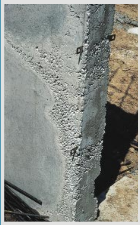
Figure 9. Concrete that's very flowable eases the labor of placement, but can cause quality concerns. Moving a wet mix too far with hoes can create segregation (left), while the increased pressure created by vibrating a wet mix may snap a form tie and "pillow out" the wall (right).
