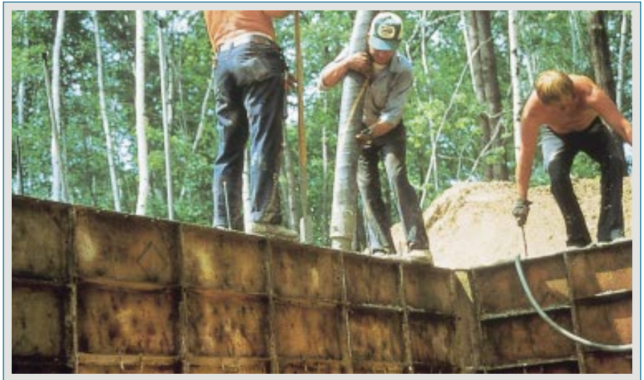
Figure 8. Concrete flowing rapidly down a chute (left) may have more added water than would be ideal. Stiff concrete can be placed more easily by pumping (below). A mechanical vibrator (bottom) is used to consolidate successive lifts.
