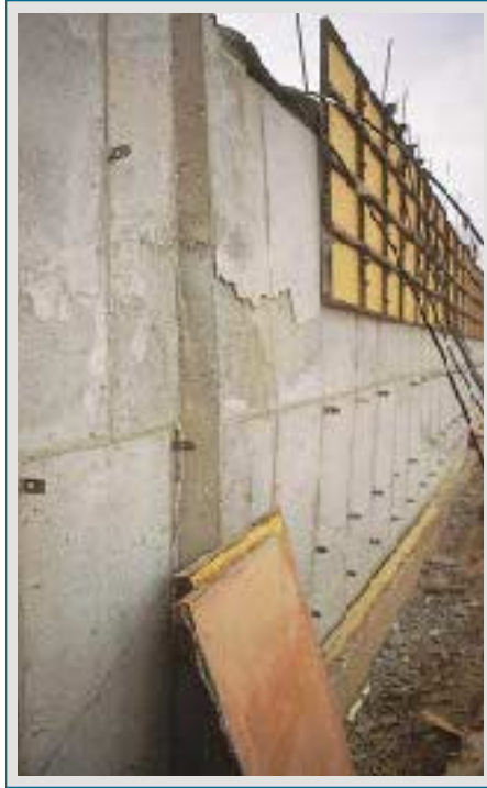
Figure 9. Concrete that's very flowable eases the labor of placement, but can cause quality concerns. Moving a wet mix too far with hoes can create segregation (left), while the increased pressure created by vibrating a wet mix may snap a form tie and "pillow out" the wall (right).
