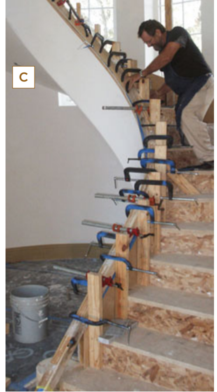
Figure 2. A bar clamp helps the author twist the rail to conform to the curb; bar clamps on the bottom and top forms prevent the rail from jumping over the forms as it is pulled into shape (A). Deep-throated C-clamps are needed to clamp the bottom of the rail to the forms (B). It takes a lot of clamps and sometimes a little bit of force to bend and twist the rail into position (C, D).
