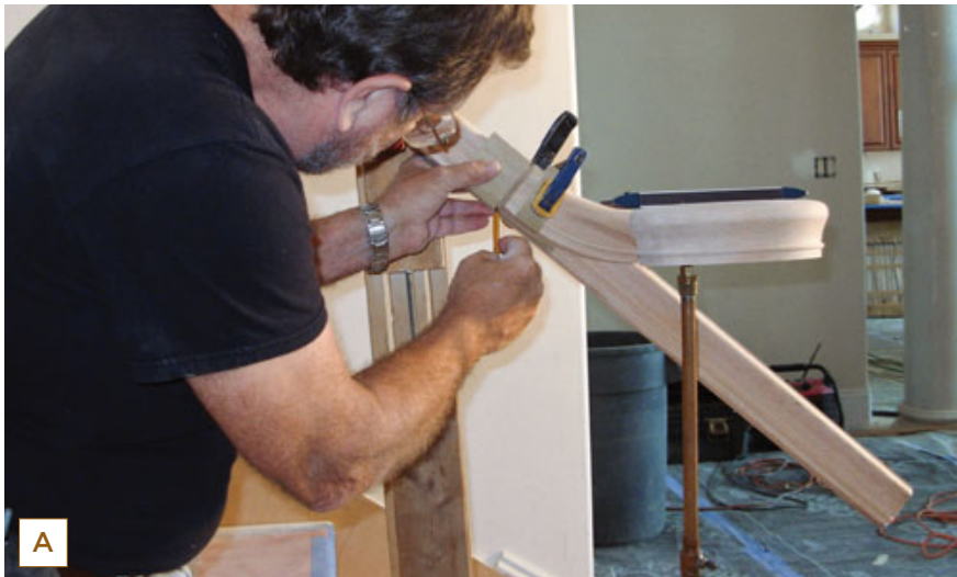
Figure 7. With the up-easing cut to the rake angle, the author plumbs the volute down to the centerline of the starter step, clamps the fitting in place, and scribes the cut on the handrail (A). A shooting board fastened to 2x4s clamped to the handrail will help guide the cut, which is made in place with a circular saw (B). Then the lower volute is fastened to the handrail with a rail bolt (C).
