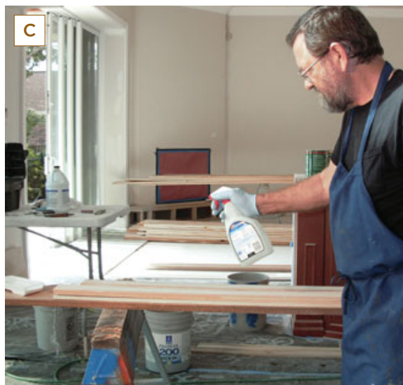
Figure 1. The author lines the bending mold with shrink-wrap to keep glue from sticking to the rail and bending mold (A). After applying an even coat of glue to each lamination with a 2-inch roller (B), the author lightly mists the glue with water (C). A few quick wraps with plastic at the ends and in the middle secures the bundle (D).
