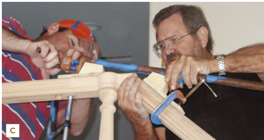
Figure 8. The handrail transitions to a 42-inch-high level balcony rail (A). After cutting the miters and fitting the newel post, the author joins the rail sections together with a small biscuit and epoxy (B). A pair of angled blocks attached to short pieces of plywood create leverage points for the pipe clamp used to draw the joint together (C).
