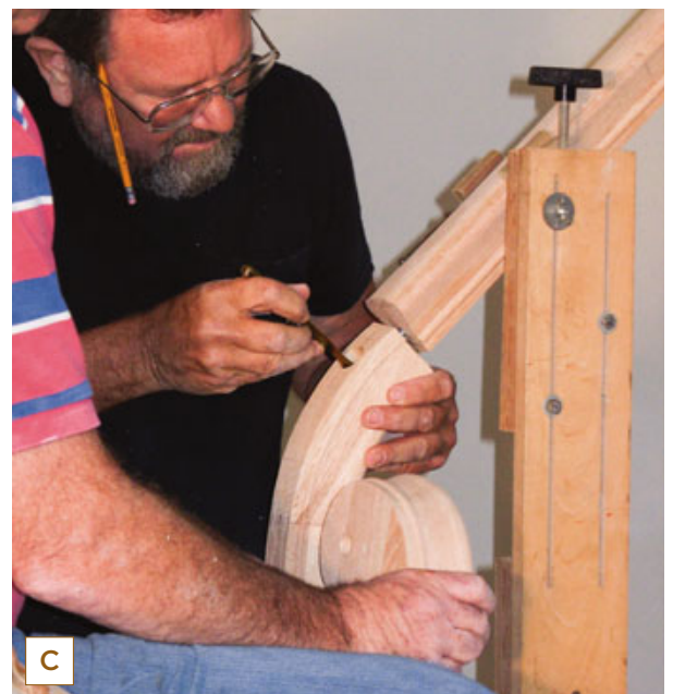
Figure 7. With the up-easing cut to the rake angle, the author plumbs the volute down to the centerline of the starter step, clamps the fitting in place, and scribes the cut on the handrail (A). A shooting board fastened to 2x4s clamped to the handrail will help guide the cut, which is made in place with a circular saw (B). Then the lower volute is fastened to the handrail with a rail bolt (C).
