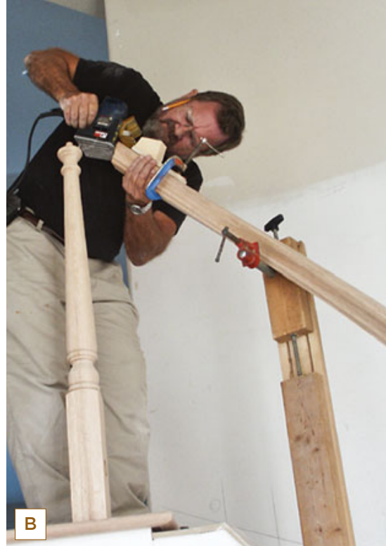
Figure 8. The handrail transitions to a 42-inch-high level balcony rail (A). After cutting the miters and fitting the newel post, the author joins the rail sections together with a small biscuit and epoxy (B). A pair of angled blocks attached to short pieces of plywood create leverage points for the pipe clamp used to draw the joint together (C).
