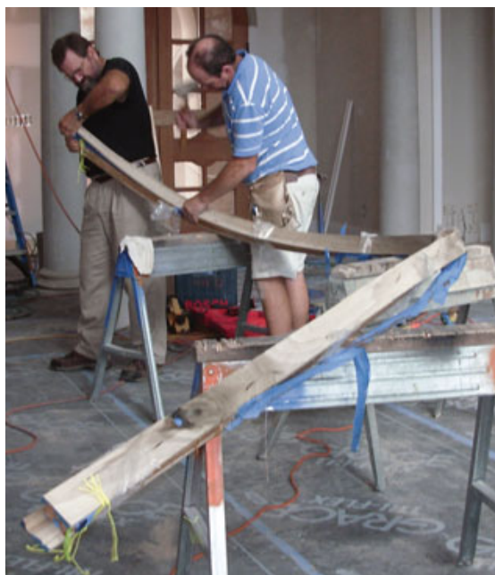
Figure 3. To minimize springback, rail sections should set at least 72 hours before they're removed from the form (left). Cleanup is done with scrapers, sanders, and Tadpole profiled sandpaper holders for the beads and hollows (below).
