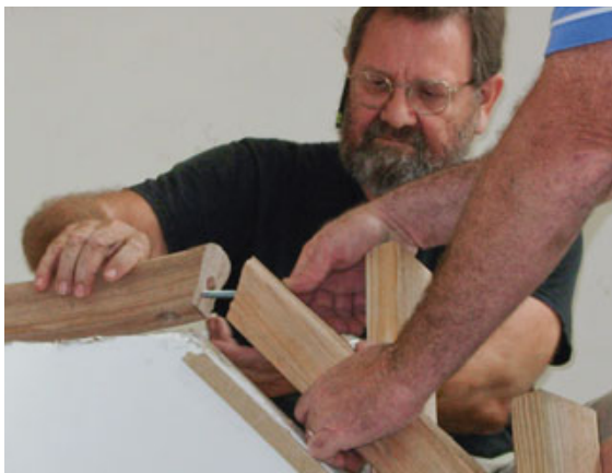
Figure 5. The lower, middle, and upper rail sections are bolted together with rail bolts, but the author won't glue the joints until the entire rail has been positioned and the lower volute and upper tandem cap have been installed.
