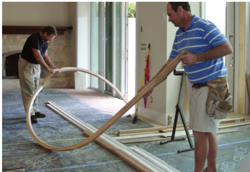
Figure 5. The lower, middle, and upper rail sections are bolted together with rail bolts, but the author won't glue the joints until the entire rail has been positioned and the lower volute and upper tandem cap have been installed.
