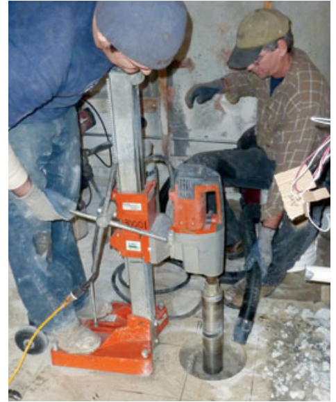
Figure 2. Once the floor was mapped, plumbers drilled holes in the slab to move supply and DWV lines to their new locations.
