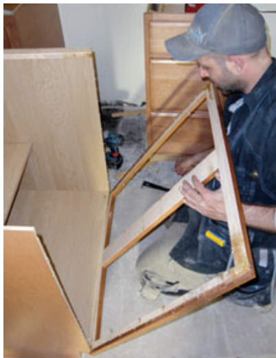
Figure 6. The author ordered face-frame and door assemblies sized to fit vanity cabinets and in a finish that matched the kitchen cabinets, then applied them to stock boxes that had been modified to fit under a 34-inch-high countertop.
