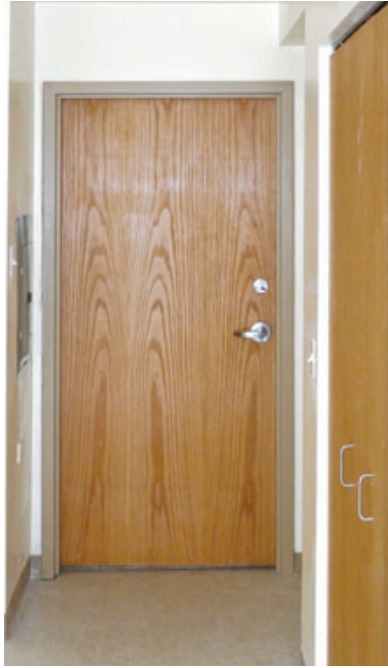
Figure 5. All of the doorways needed to be widened to a full 3/0 to accommodate a wheelchair (far left). Though the location of an existing drain made it impossible to provide a full 5-foot clear floor space at the entry inside the apartment (left), HUD rules permit the clearance to be outside the apartment in the hallway (above).
