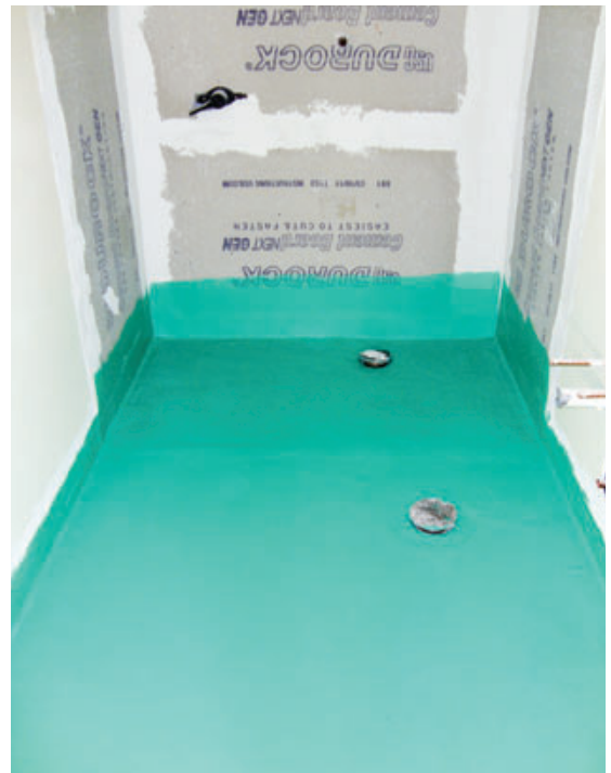
Figure 4. The original shower base had a 3-inch-high curb, common in standard construction but a major obstacle to a wheelchair (above). After removing it, the author lowered the concrete slab in the shower area by an inch, smoothed and sloped the surface toward the new drain, and waterproofed the entire bathroom floor with a liquid waterproofing membrane (right).
