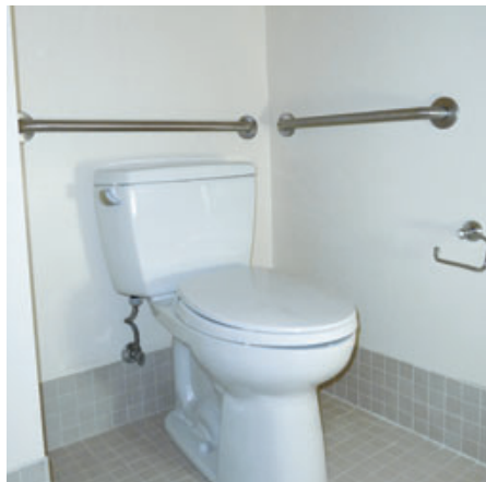
Figure 8. The barrier-free shower is equipped with a flexible rubber dam that helps contain water without inhibiting wheelchair access; note the second floor drain under the sink (below). Like the shower, the high-rise toilet is equipped with grab bars securely fastened to wood blocking (left).
