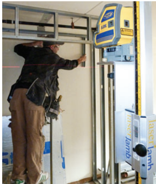
Figure 3. With no structural loads to worry about, the new partition walls were quickly framed with steel studs (left). Plenty of blocking was needed to easily position and install grab bars, a fold-down shower seat, and other accessories (below).
