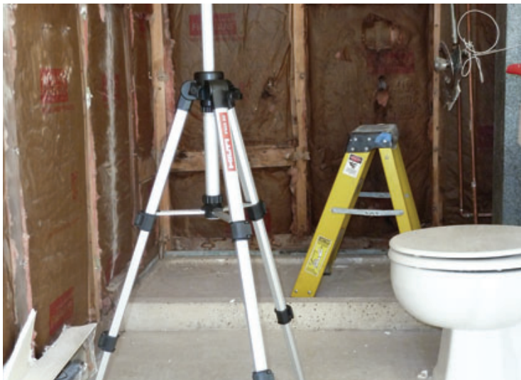
Figure 4. The original shower base had a 3-inch-high curb, common in standard construction but a major obstacle to a wheelchair (above). After removing it, the author lowered the concrete slab in the shower area by an inch, smoothed and sloped the surface toward the new drain, and waterproofed the entire bathroom floor with a liquid waterproofing membrane (right).
