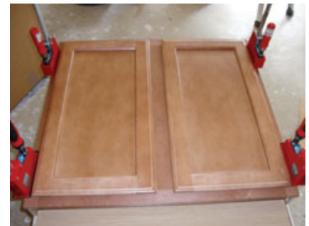
Figure 6. The author ordered face-frame and door assemblies sized to fit vanity cabinets and in a finish that matched the kitchen cabinets, then applied them to stock boxes that had been modified to fit under a 34-inch-high countertop.
