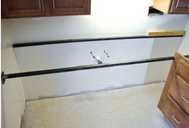
Figure 7. The sink countertop is supported by steel angle at the wall and bar stock at the front (left), so that the cabinets underneath can be quickly removed for wheelchair access without interfering with the countertop or plumbing (right).
