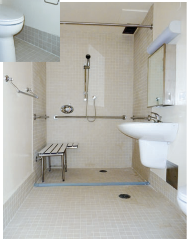
Figure 8. The barrier-free shower is equipped with a flexible rubber dam that helps contain water without inhibiting wheelchair access; note the second floor drain under the sink (below). Like the shower, the high-rise toilet is equipped with grab bars securely fastened to wood blocking (left).
