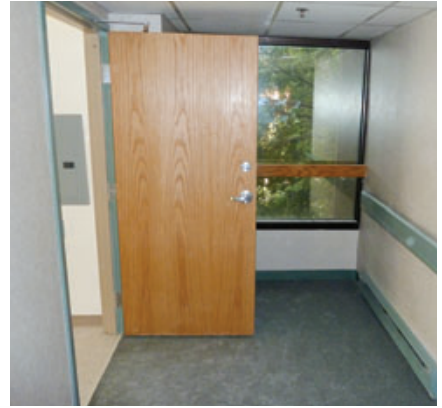
Figure 5. All of the doorways needed to be widened to a full 3/0 to accommodate a wheelchair (far left). Though the location of an existing drain made it impossible to provide a full 5-foot clear floor space at the entry inside the apartment (left), HUD rules permit the clearance to be outside the apartment in the hallway (above).
