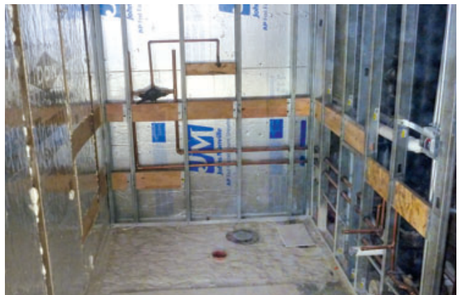
Figure 3. With no structural loads to worry about, the new partition walls were quickly framed with steel studs (left). Plenty of blocking was needed to easily position and install grab bars, a fold-down shower seat, and other accessories (below).
