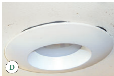
Figure 8. A strip of foil tape seals an air leak in an “airtight” ceiling can (A). The much larger — and often overlooked — leak between the fixture and the ceiling drywall has been sealed with tape (B). On a can with an integral trim ring that prevents the use of tape, a rolled “shoelace” of duct putty forms a seal (C). Excess putty that squeezes out is removed later (D).
