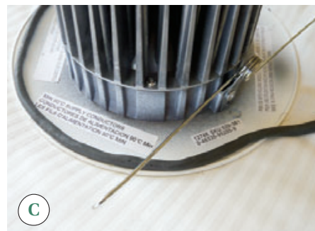
Figure 8. A strip of foil tape seals an air leak in an “airtight” ceiling can (A). The much larger — and often overlooked — leak between the fixture and the ceiling drywall has been sealed with tape (B). On a can with an integral trim ring that prevents the use of tape, a rolled “shoelace” of duct putty forms a seal (C). Excess putty that squeezes out is removed later (D).
