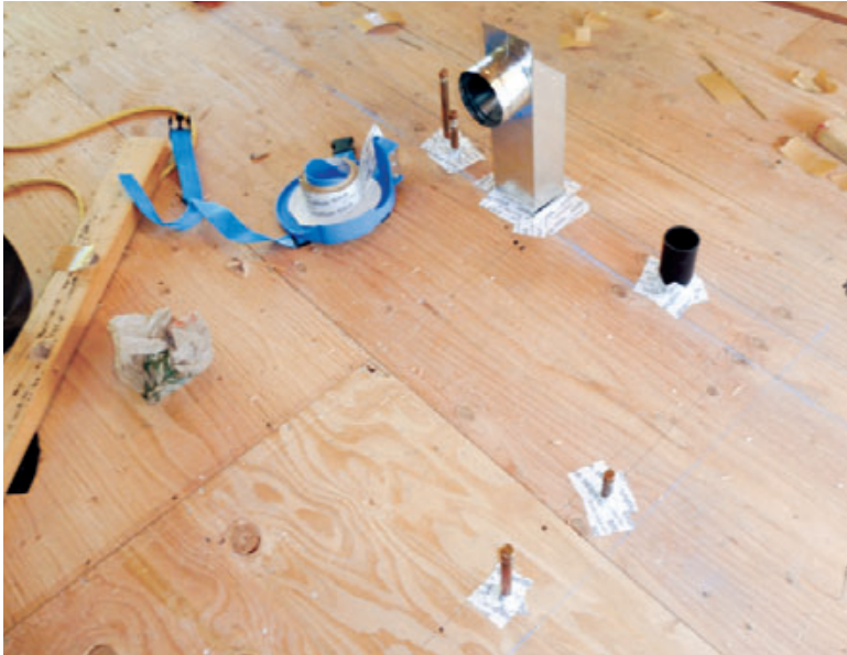
Figure 3. Floor penetrations that will be enclosed in a partition wall are best sealed at the level of the subfloor (left), rather than where they pass through the plate. In retrofit applications where that's not an option, air leakage under the plate can be reduced by sealing the area with duct mastic (above).
