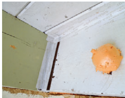
Figure 11. Plywood bedded in polyurethane foam seals air leaks between blocking and rafter tails. A stucco wall finish will cover the raw bottom edge of the plywood (above). A nearby rafter bay has been sealed with tape instead of foam — a time-consuming but more positive solution. The excess foam that marks an injection hole for dense-pack cellulose will be trimmed off, and the tape covered with a plywood trim piece, as above (left).
