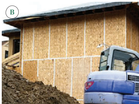
Figure 9. When wall sheathing is set in beads of polyurethane foam, temporary blocks at the base make it easier to position the sheet without smearing the sealant (A). For extra insurance, seams between panels are also sealed with tape (B). An intentional 1/4-inch gap below the drywall on exterior walls is easily filled with canned foam (C). In a retrofit project, it’s a good idea to protect the finish floor with paper or tape first.
