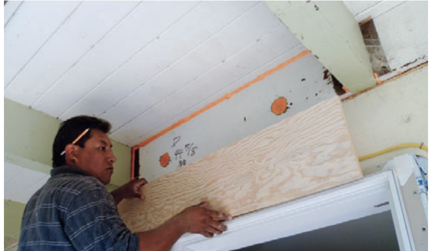
Figure 11. Plywood bedded in polyurethane foam seals air leaks between blocking and rafter tails. A stucco wall finish will cover the raw bottom edge of the plywood (above). A nearby rafter bay has been sealed with tape instead of foam — a time-consuming but more positive solution. The excess foam that marks an injection hole for dense-pack cellulose will be trimmed off, and the tape covered with a plywood trim piece, as above (left).
