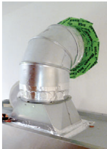
Figure 2. Small-diameter pipe penetrations through drywall or plywood are efficiently sealed with two short pieces of tape (left). Larger pipes, like this range-hood exhaust vent, may require a dozen pieces or more (right).
