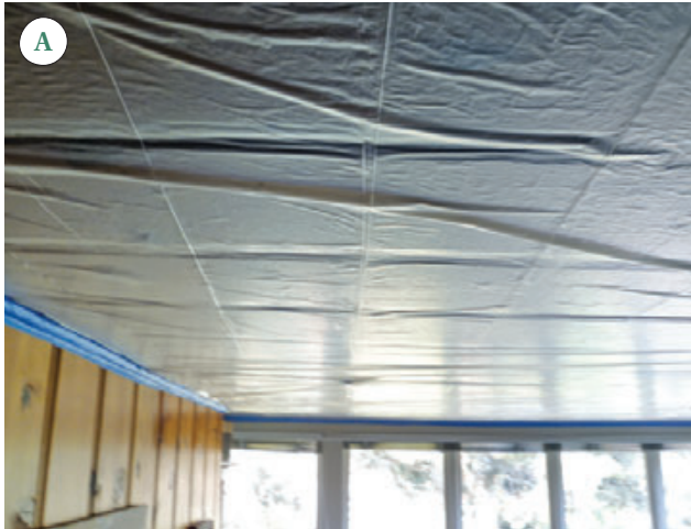
Figure 10. Warm air venting from the attic above sucks a protective plastic sheet against this single-layer T&G ceiling, illustrating its extreme permeability to moving air (A). To stop air penetration at the gable overhang of a T&G cathedral ceiling, a \frac{3}{4} -inch bit is used to bore holes where the boards cross the outermost pair of rafters (B). The holes are then injected with foam (C).
