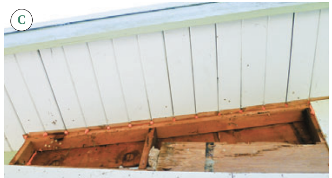
Figure 10. Warm air venting from the attic above sucks a protective plastic sheet against this single-layer T&G ceiling, illustrating its extreme permeability to moving air (A). To stop air penetration at the gable overhang of a T&G cathedral ceiling, a \frac{3}{4} -inch bit is used to bore holes where the boards cross the outermost pair of rafters (B). The holes are then injected with foam (C).
