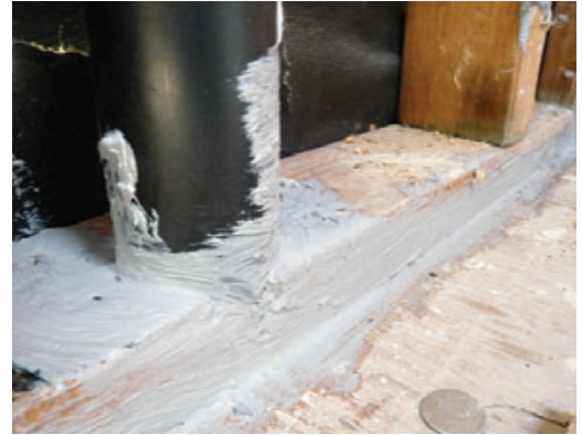
Figure 3. Floor penetrations that will be enclosed in a partition wall are best sealed at the level of the subfloor (left), rather than where they pass through the plate. In retrofit applications where that's not an option, air leakage under the plate can be reduced by sealing the area with duct mastic (above).
