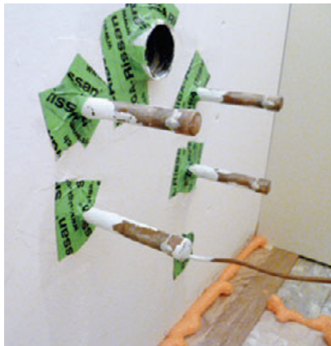
Figure 2. Small-diameter pipe penetrations through drywall or plywood are efficiently sealed with two short pieces of tape (left). Larger pipes, like this range-hood exhaust vent, may require a dozen pieces or more (right).
