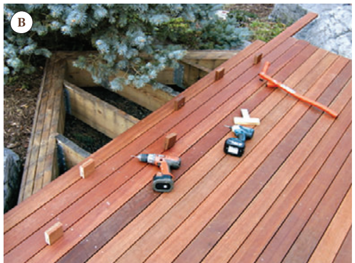
Figure 5. Jigs made with hardwood scraps and aluminum stock (A) sped up accurate drilling and spacing of deck boards. In combination with the use of a BoWrench, the spacers ensured near perfect spacing (B,C).
