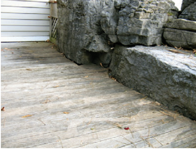
Figure 1. The surface of the 15-year-old deck was weathered and rough, and the nails were lifting out. On removing the old material, the author found that the framing was in good shape and accurately laid out.
