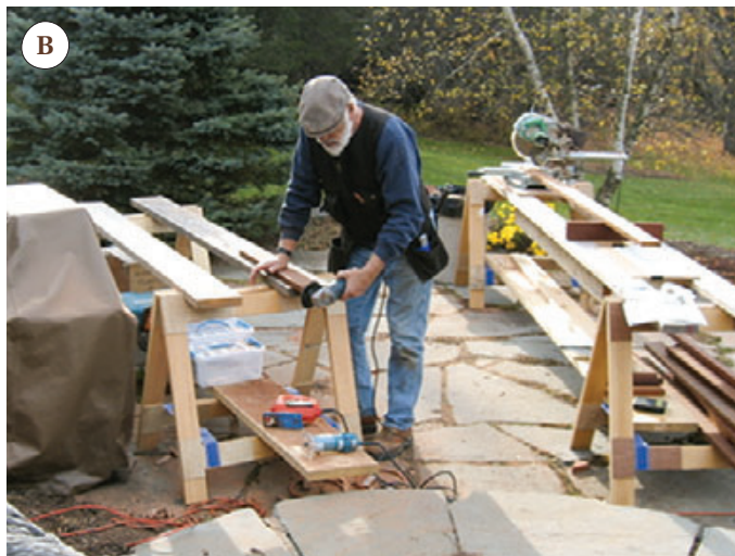
Figure 4. On site, the author used a couple of knock-down work surfaces for final trimming and scribing (A, B). The butt joints between individual deck boards were cut in the shop and the courses labeled and bundled for quick placement (C).
