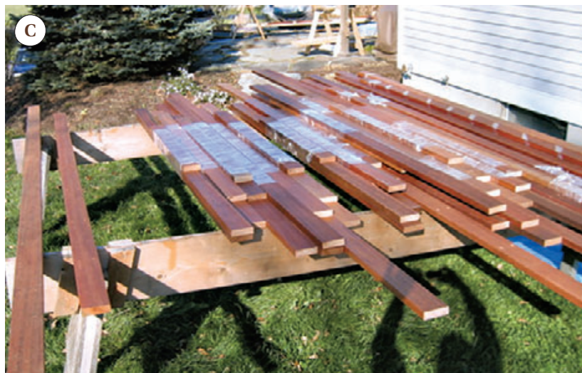
Figure 4. On site, the author used a couple of knock-down work surfaces for final trimming and scribing (A, B). The butt joints between individual deck boards were cut in the shop and the courses labeled and bundled for quick placement (C).
