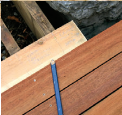
Figure 2. Using 1x4s as story poles allowed the author to take the exact joist layout back to the shop where he could accurately cut the decking.
