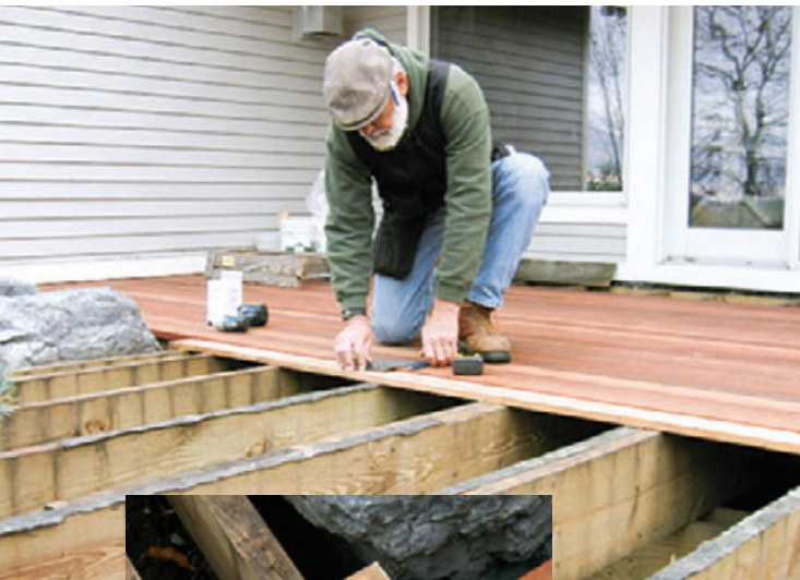
Figure 2. Using 1x4s as story poles allowed the author to take the exact joist layout back to the shop where he could accurately cut the decking.
