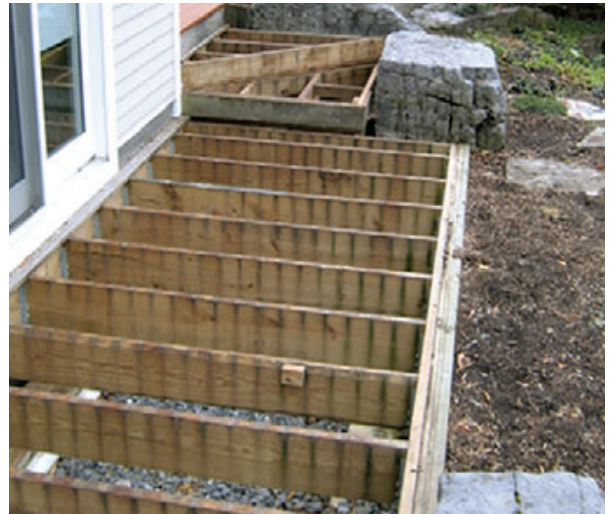
Figure 1. The surface of the 15-year-old deck was weathered and rough, and the nails were lifting out. On removing the old material, the author found that the framing was in good shape and accurately laid out.
