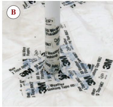
Figure 2. A sheet of 10-mil poly, which acts as an air and vapor barrier and a capillary break, was laid on top of the EPS (A); all seams and penetrations were sealed with 3M flashing tape (B). Steel rebar and wire mesh were supported on dobies cut from insulation scraps (C). Because it is also the finished floor, the slab was meticulously power-troweled smooth and flat (D).
