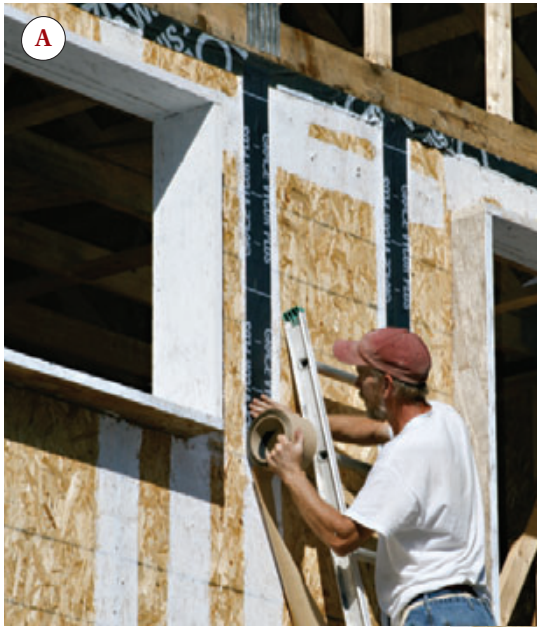
Figure 6. Sealing the sheathing with flashing tape created the building's airtight envelope (A). The exposed outer face of the forms was protected with Durock and a cementitious parge (B); its top was covered with asphalt-coated fiberboard sheathing and aluminum flashing (C).
