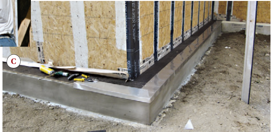
Figure 6. Sealing the sheathing with flashing tape created the building's airtight envelope (A). The exposed outer face of the forms was protected with Durock and a cementitious parge (B); its top was covered with asphalt-coated fiberboard sheathing and aluminum flashing (C).
