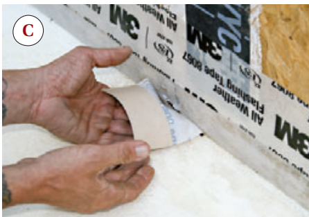
Figure 5. To make a tight seal between the subslab poly barrier and the sheathing, the author first taped the corner of the plastic sheet to the OSB (A), then folded it up onto the wall (B). The edge of the plastic sheet was continuously taped, and all holes carefully sealed (C,D).
