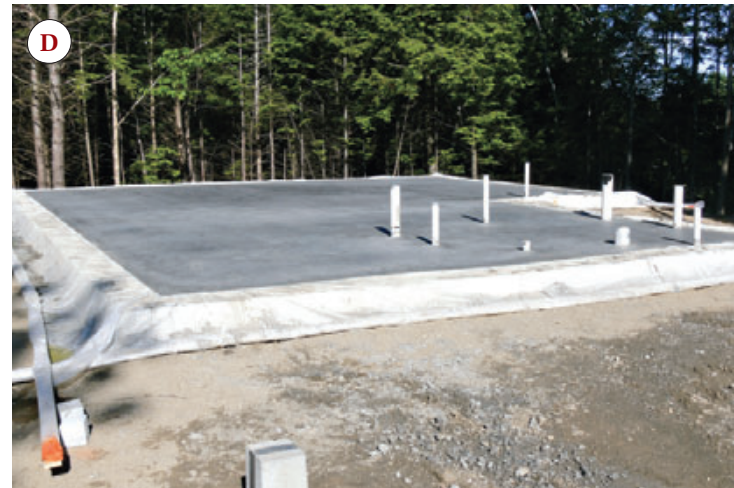
Figure 2. A sheet of 10-mil poly, which acts as an air and vapor barrier and a capillary break, was laid on top of the EPS (A); all seams and penetrations were sealed with 3M flashing tape (B). Steel rebar and wire mesh were supported on dobies cut from insulation scraps (C). Because it is also the finished floor, the slab was meticulously power-troweled smooth and flat (D).
