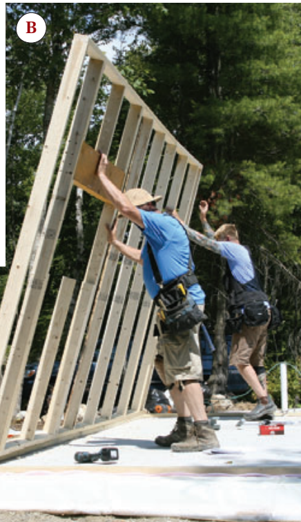
Figure 3. To protect the poly air barrier, the crew rolled out sill seal (A) before standing the conventionally framed inner 2x4 support walls (B). The walls were anchored to the slab (C), and the drilled holes sealed with spray foam (D).
