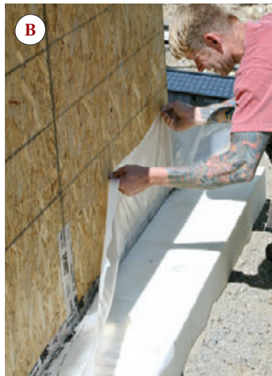
Figure 4. After pulling back the poly vapor barrier, the crew installed the OSB sheathing over beads of spray foam.
