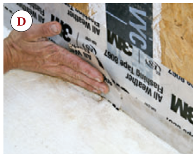
Figure 5. To make a tight seal between the subslab poly barrier and the sheathing, the author first taped the corner of the plastic sheet to the OSB (A), then folded it up onto the wall (B). The edge of the plastic sheet was continuously taped, and all holes carefully sealed (C,D).
