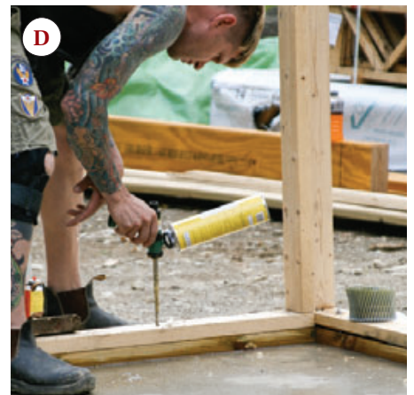
Figure 3. To protect the poly air barrier, the crew rolled out sill seal (A) before standing the conventionally framed inner 2x4 support walls (B). The walls were anchored to the slab (C), and the drilled holes sealed with spray foam (D).
