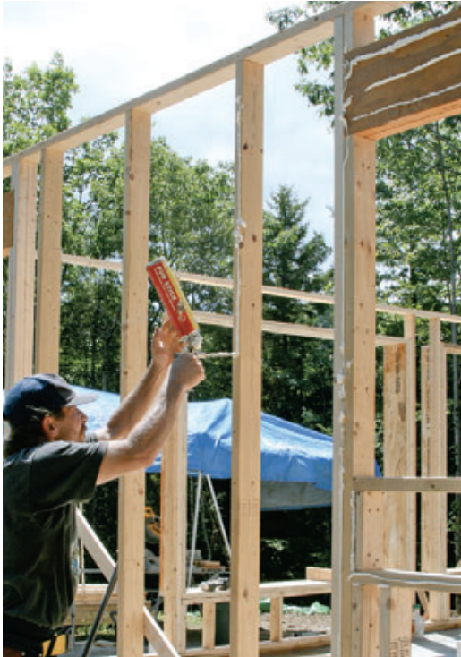
Figure 4. After pulling back the poly vapor barrier, the crew installed the OSB sheathing over beads of spray foam.
