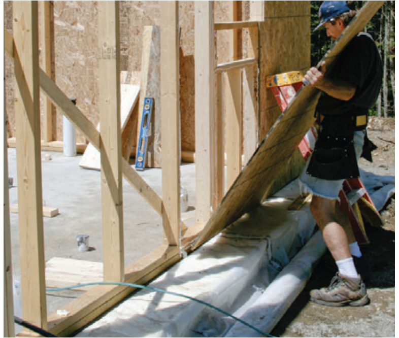
Figure 4. After pulling back the poly vapor barrier, the crew installed the OSB sheathing over beads of spray foam.
