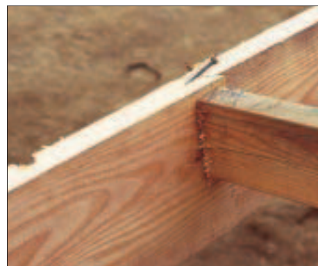
Figure 2. To cut a mitered lap joint, the author scribes a line on the back side of the uncut fascia and, with the saw set at 45 degrees, makes the cut from the outside face of the board, making sure the blade follows the scribe line (left). An angled nail driven into the top edge of mating board provides a third hand for hanging the next piece (above).
