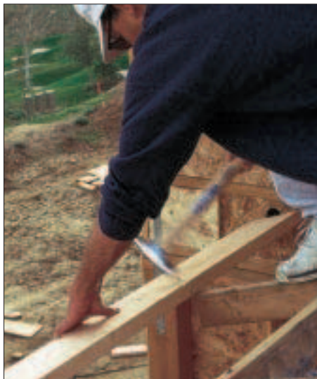
Figure 1. To hang a long piece of fascia by himself, the author makes the first cut from the roof as the fascia leans against the building (top left). He then lays the board across the rafter tails, finish side down. Working near one end, he drives a nail at an angle until the point protrudes 1/4 inch from the back side (top right). He moves the fascia out to the edge and drives that nail into the top of the plumb cut of the rafter tail (above left). Moving to the other end, he swings the board down into place (above right) and nails it off.
