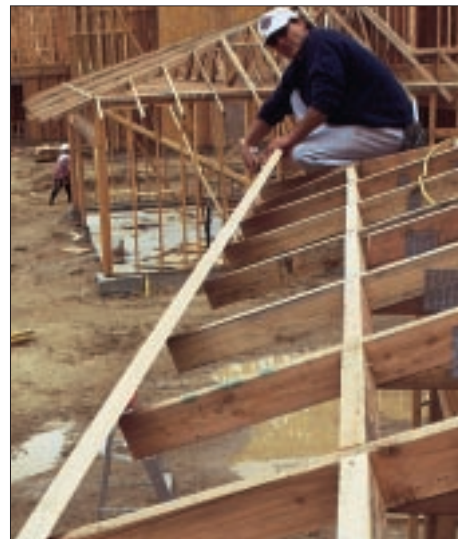
Figure 1. To hang a long piece of fascia by himself, the author makes the first cut from the roof as the fascia leans against the building (top left). He then lays the board across the rafter tails, finish side down. Working near one end, he drives a nail at an angle until the point protrudes 1/4 inch from the back side (top right). He moves the fascia out to the edge and drives that nail into the top of the plumb cut of the rafter tail (above left). Moving to the other end, he swings the board down into place (above right) and nails it off.
