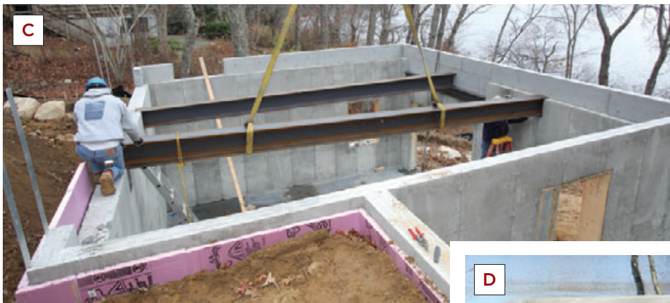
Figure 2. I-beams provide midspan support for the garage floor. A header beam spans the door opening at the rear of the building (A) and also supports one of the I-beams (B). The second beam sits in the formed foundation pockets (C). Sections of steel channel shimmed to the correct elevation on top of the header support the perimeter steel angle (D).
