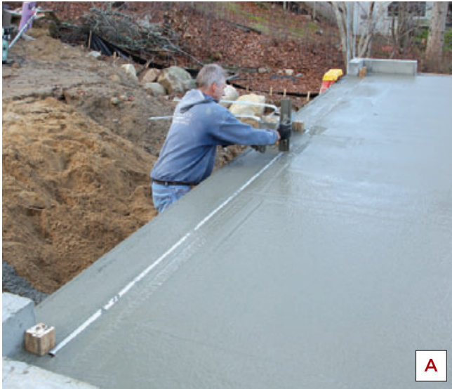
Figure 5. To create a weather lip at the garage doors, the foundation contractor sinks a length of galvanized pipe into the wet concrete (A), then finishes the sloping apron in front (B). The pipe creates a gentle but durable transition from the apron to the floor inside (C). The finished garage blends neatly into the hillside (D).
