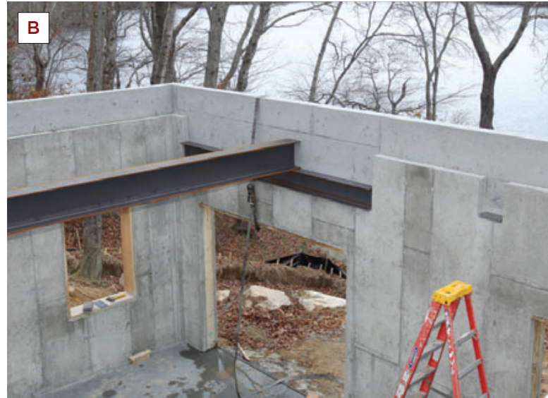
Figure 2. I-beams provide midspan support for the garage floor. A header beam spans the door opening at the rear of the building (A) and also supports one of the I-beams (B). The second beam sits in the formed foundation pockets (C). Sections of steel channel shimmed to the correct elevation on top of the header support the perimeter steel angle (D).
