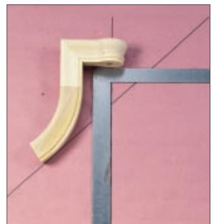
**Figure 6.** Use the same process to find the height of the landing newel and mark the cut on the gooseneck.
