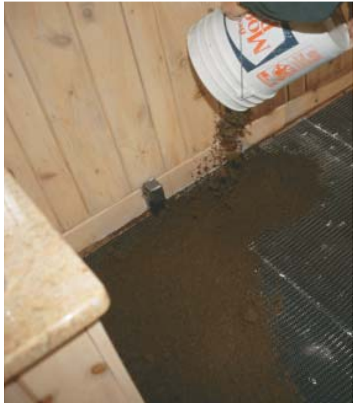
Figure 3. The mud mix, or “screed” — a combination of Portland cement, sand, and water — is mixed fairly dry, so that it holds its shape when compressed (above). The mix is first dumped around the perimeter of the room to establish screeding points for leveling the general floor area (right).
