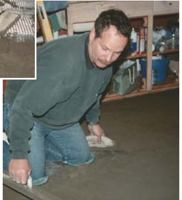
Figure 5. The author floats the floor by adding mix between lines and leveling it with a straightedge. The mud is packed and floated in one two-fisted action: A wood trowel levels and fills the base, followed by a steel float for a smooth finish.
