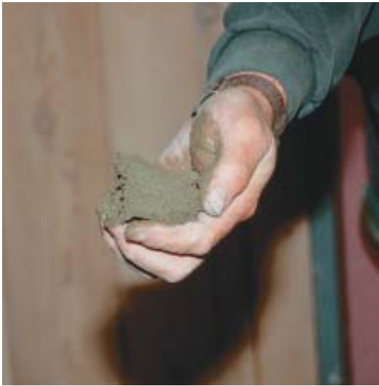
Figure 3. The mud mix, or “screed” — a combination of Portland cement, sand, and water — is mixed fairly dry, so that it holds its shape when compressed (above). The mix is first dumped around the perimeter of the room to establish screeding points for leveling the general floor area (right).
