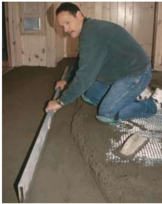
Figure 5. The author floats the floor by adding mix between lines and leveling it with a straightedge. The mud is packed and floated in one two-fisted action: A wood trowel levels and fills the base, followed by a steel float for a smooth finish.
