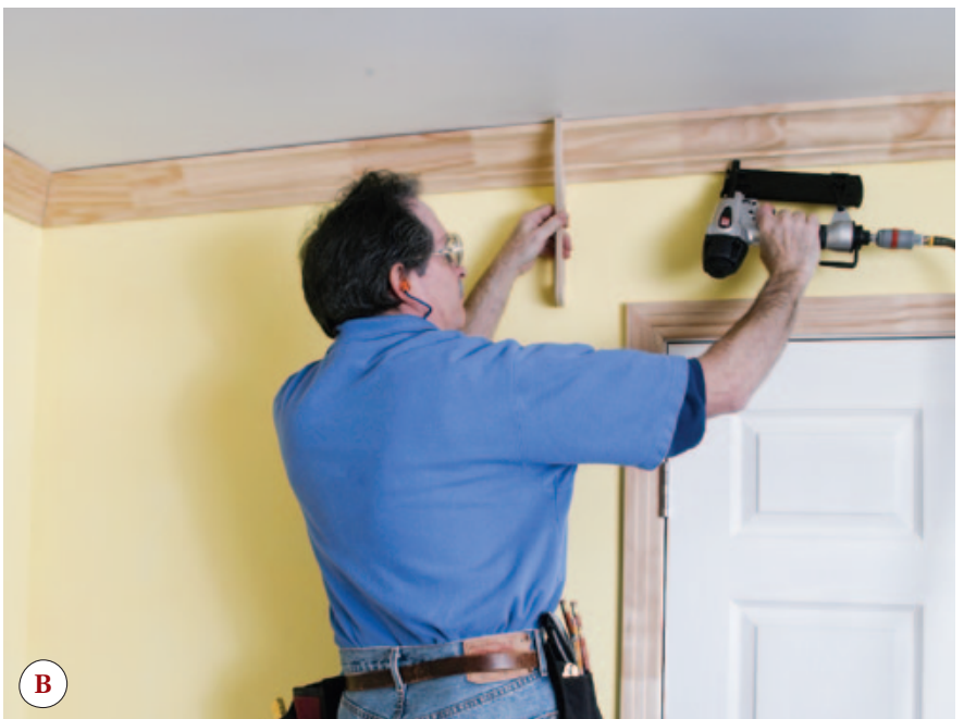
Figure 13. The end of the piece shown in Figure 12 is aligned with the layout marks on the wall (A) to ensure that the coped end of the next piece (B) fits snugly, with no need for fine-tuning the joint.
