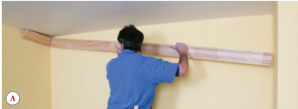
Figure 10. The coped end of the first piece of crown is snugged against the starter piece (A). The author fastens only the right half of that piece so that it can be flexed away from the wall when the last piece slips in (B).
