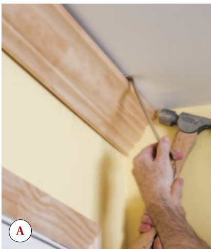
Figure 13. The end of the piece shown in Figure 12 is aligned with the layout marks on the wall (A) to ensure that the coped end of the next piece (B) fits snugly, with no need for fine-tuning the joint.
