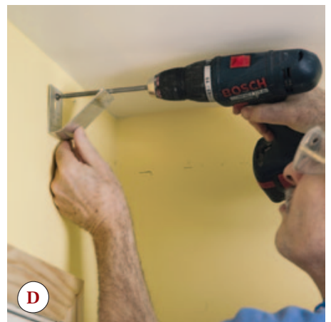
Figure 7. When working without a helper, the author uses a crown hook (A). The jig is easy to make from a scrap of sheet metal: Drill a keyhole (B) and bend the metal (C). Install the hook with a loosely driven screw placed so that it won't interfere with the crown (D).
