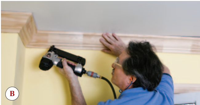
Figure 12. When working solo, the author uses his crown hook to support one end of the molding (A). He starts fastening at the coped end (B), then moves to the center of the wall, using the crown holder for accurate placement (C).
