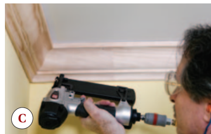
Figure 15. Finally, the still-unattached coped end of the first piece is snugged into place (A) and nailed off (B, C).
