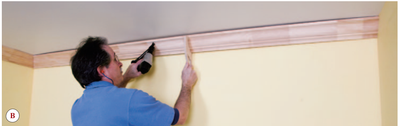
Figure 10. The coped end of the first piece of crown is snugged against the starter piece (A). The author fastens only the right half of that piece so that it can be flexed away from the wall when the last piece slips in (B).
