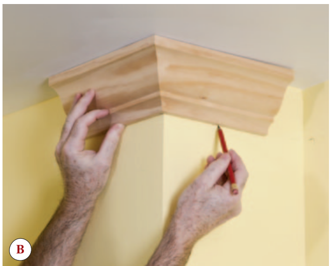
Figure 8. Using a corner mockup (A) to lay out outside corners (B) saves time when cutting the joints.
