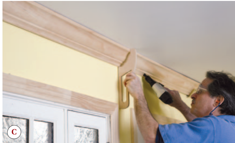
Figure 12. When working solo, the author uses his crown hook to support one end of the molding (A). He starts fastening at the coped end (B), then moves to the center of the wall, using the crown holder for accurate placement (C).
