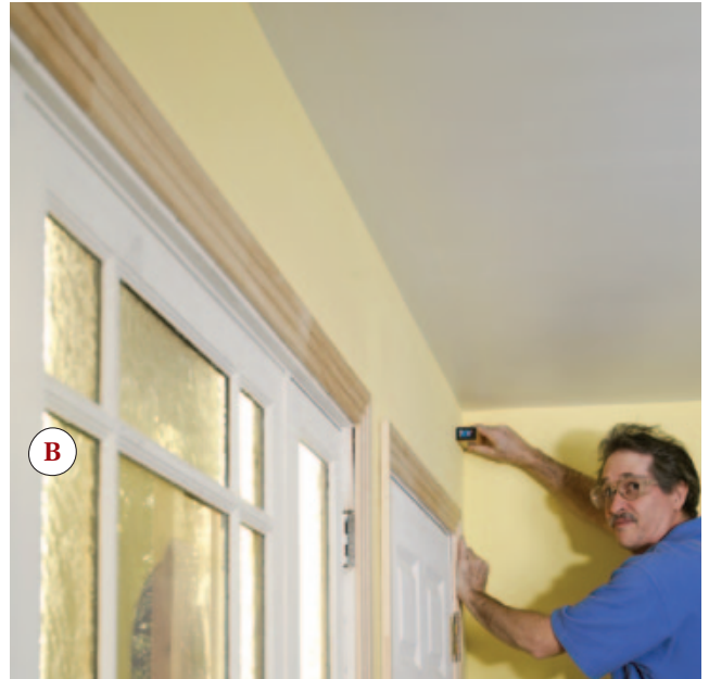
Figure 1. A tape works fine for shorter measurements (A), but a laser measurer makes it easy to measure two long walls from a single ladder setup (B). The author records measurements in a logical order as he works around the room (C).
