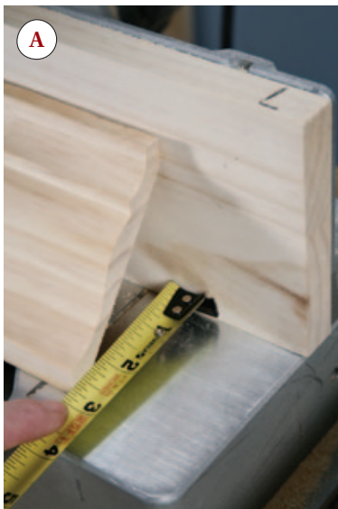
Figure 2. With the crown upside-down, the author measures its horizontal projection (A), then rips a gauge block that width to use in setting the crown stop (B).
