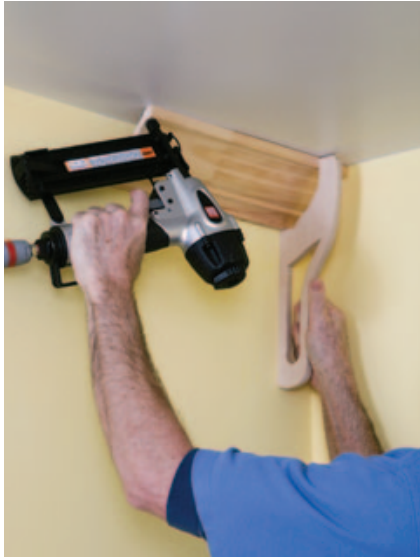
Figure 9. The author works around the room from left to right, with copes on the left ends and butt cuts on the right. The process starts with a temporary starter piece carefully positioned and tacked into place in the corner of the last wall (photo, above).
