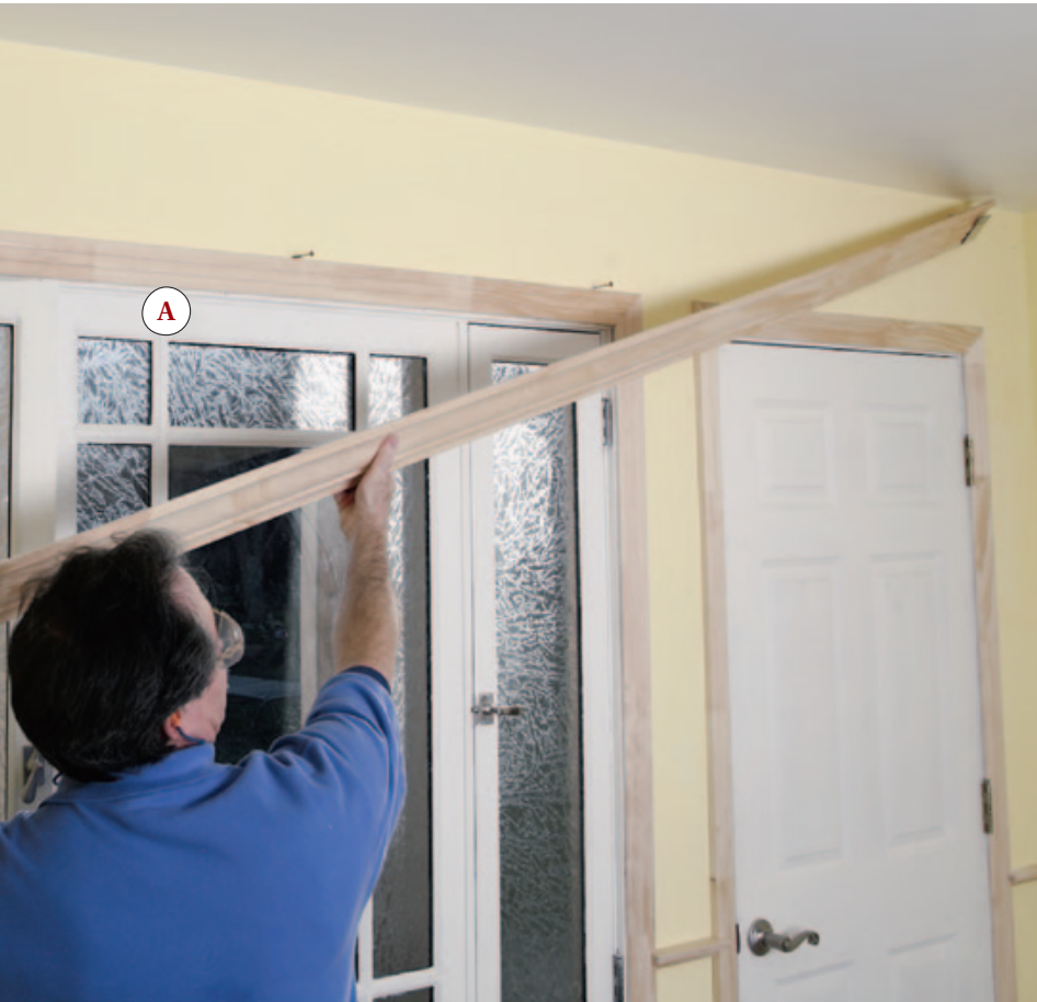
Figure 7. When working without a helper, the author uses a crown hook (A). The jig is easy to make from a scrap of sheet metal: Drill a keyhole (B) and bend the metal (C). Install the hook with a loosely driven screw placed so that it won't interfere with the crown (D).
