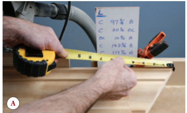
Figure 4. After measuring and cutting a coped end to length (A), the author cuts off the tip before removing the piece from the saw (B). When cutting outside corners (C), he pulls the measurement from the auxiliary fence, with the short point of the miter flush with the fence.
