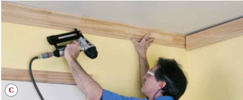
Figure 14. When the author reaches the last wall, he removes the temporary starter piece (A), then flexes the first piece away from the wall with his right hand while supporting the last piece in his left hand (B). He slips the last piece in behind the coped end of the first piece and nails it off (C).
