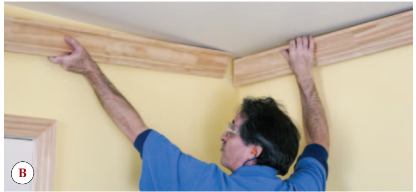
Figure 14. When the author reaches the last wall, he removes the temporary starter piece (A), then flexes the first piece away from the wall with his right hand while supporting the last piece in his left hand (B). He slips the last piece in behind the coped end of the first piece and nails it off (C).
