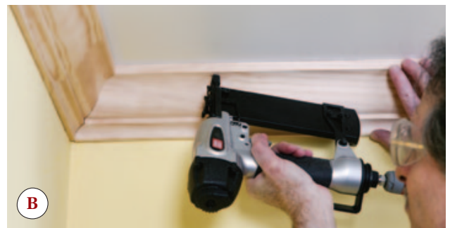
Figure 15. Finally, the still-unattached coped end of the first piece is snugged into place (A) and nailed off (B, C).
