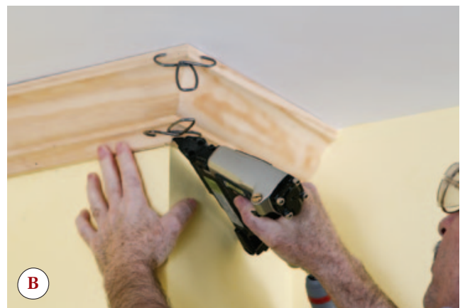
Figure 11. Outside corners are gently tacked so the miter can be adjusted if needed (A). The author glues and spring-clamps the joint to ensure it never opens up (B).
