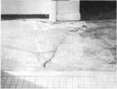
Cement-based toppings are strong and stiff, and can go on as thin as 1/8 inch—making them ideal for slab repair. Over wood substrates, they require metal lath.
