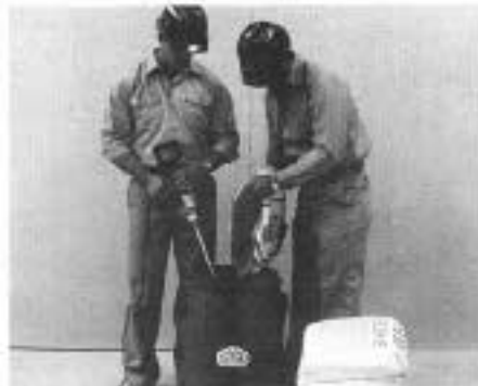
For small jobs, cement-based toppings such as Quikrete or Ardex can be mixed on site with a 1/2-inch drill and paddle (left) and poured into place (right). Maximum thickness is 1 inch, unless aggregate is added.
