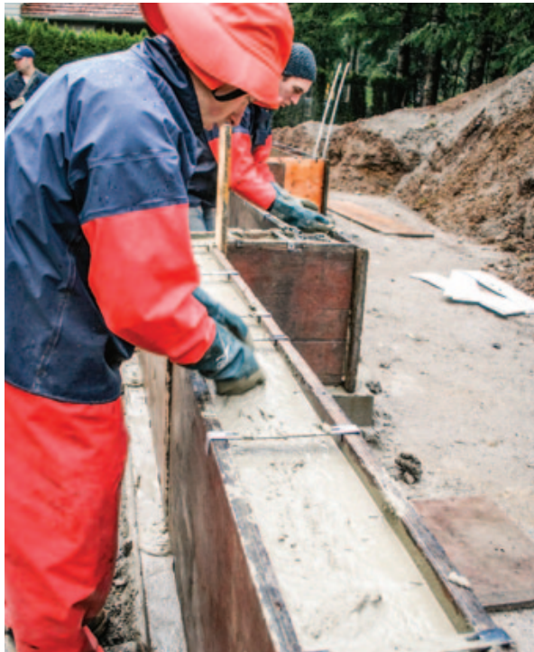
Figure 4. The author forms 8-foot-tall walls vertically, placing snap ties in slots located 1, 2, 4, 6, and 7 feet along the panel edges.
