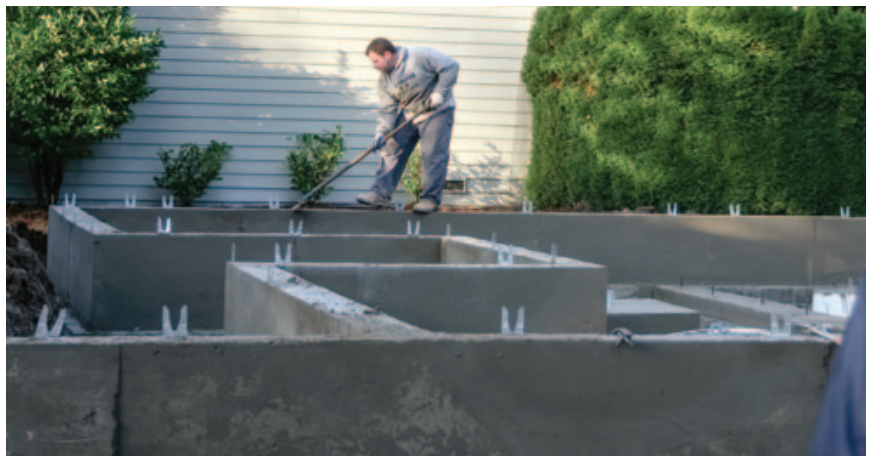
Figure 9. Before installing the mudsills, the author uses a scraper to smooth out any trowelling irregularities on the top of the stem walls.
