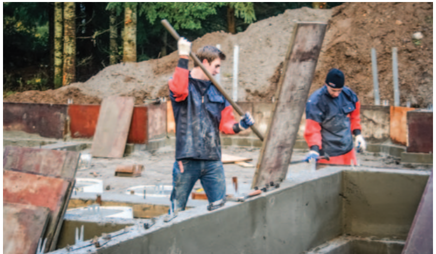
Figure 8. Workers scrape the panels clean as they strip the forms from the foundation. Later, they'll oil the panels before storing them.
