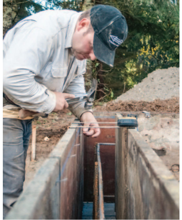
Figure 5. A reference line snapped within the top inch or two of the forms indicates the elevation of the top of the wall. The author tacks a 3d finish nail every 12 to 16 inches along the snapped lines to make them easier to find during the pour.
